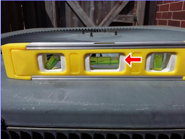
B. Item 9(Picture) unit 2 for the home not level Has been leveled
