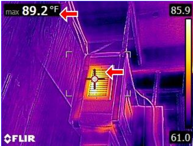
A. Item 3(Picture) 1st floor garage
