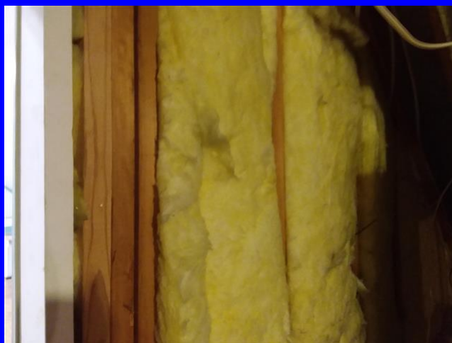
garage attic insulation
