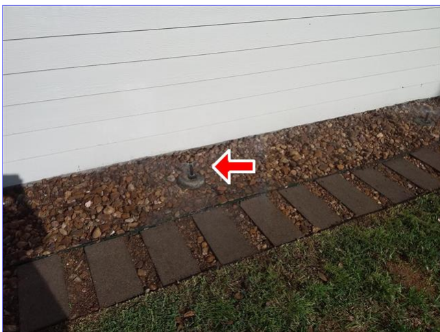
A. Item 3(Picture) zone 7 leak Repaired
