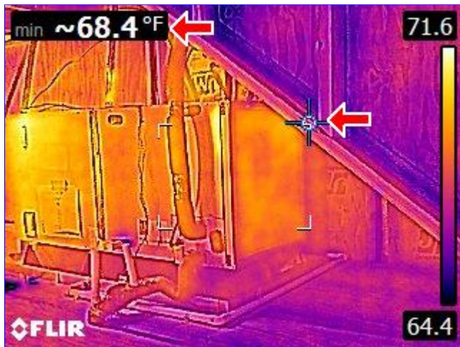
B. Item 6(Picture) 1st floor garage
