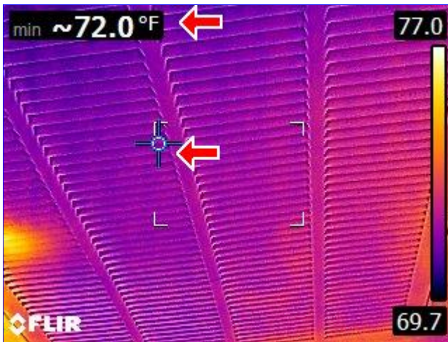
B. Item 4(Picture) 2nd floor
