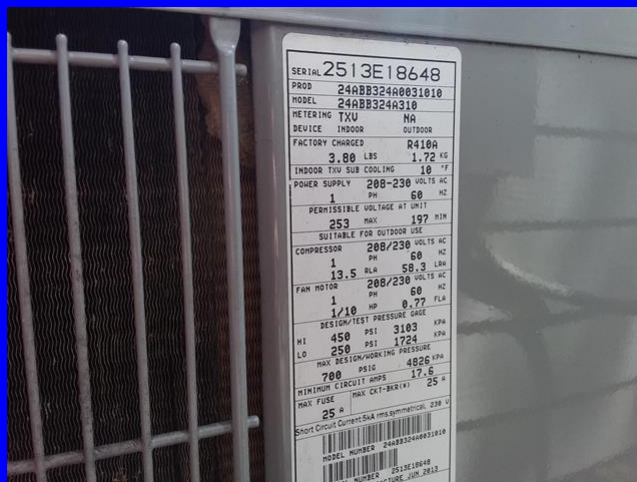
garage unit 2 label
