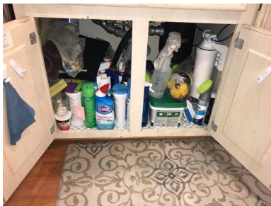
General Photos of Range Hood/Exhaust Systems:
