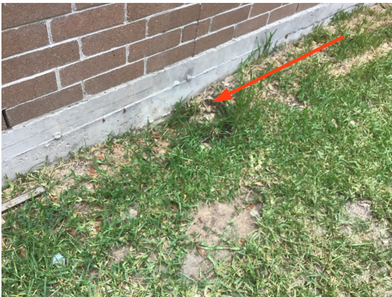
Low area next to the foundation
