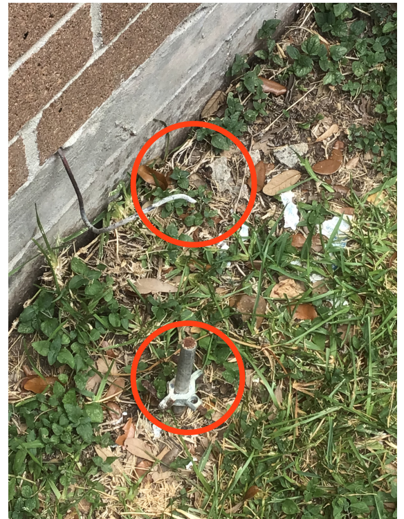
Disconnected grounding rod
