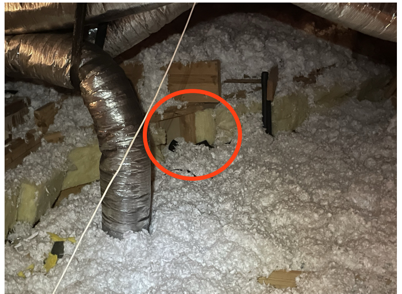
Falling insulation
