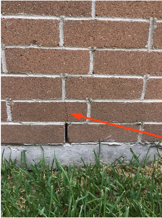
Cracks in the brick veneer
