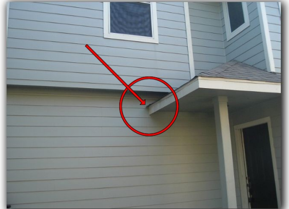
Needs kickout flashing at the front of the house
