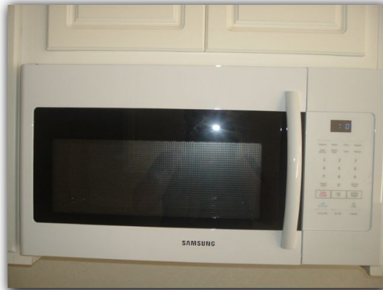
The microwave with recirculating vent performing as intended at time of the inspection.
