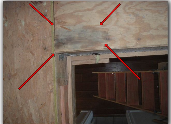
There is evidence of water penetration in the attic at the roof vent.
