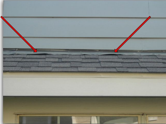
Needs kickout flashing at the front of the house
