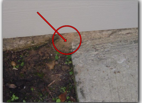
There are visible dirt tubes at the right side of the garage.
