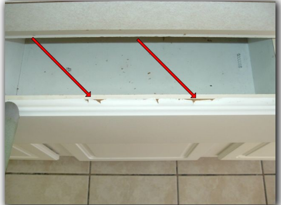
The master shower needs repair to the sealant.
