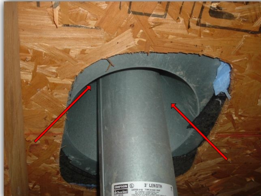
There is evidence of water penetration in the attic at the type B vent to the HVAC unit.
