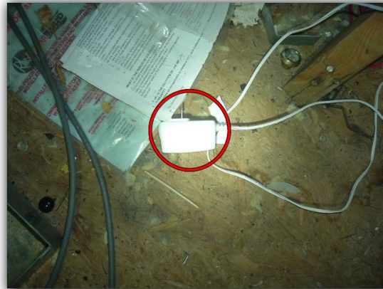
Remove the extension cord from the attic.
