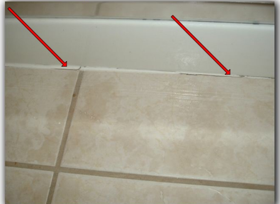
The master shower needs repair to the sealant.
