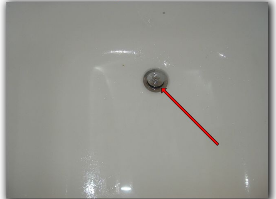
Remove the hair obstruction from the guest tub drain.
