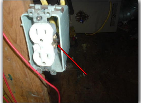
Install the cover plate at the attic receptacle
