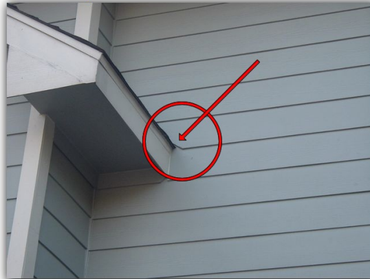
Needs kickout flashing at the front of the house
