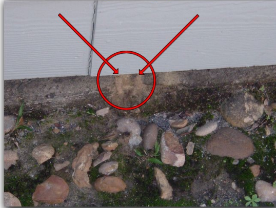
The rear exterior siding has damage.
