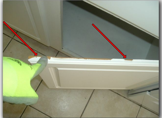
The kitchen cabinets/drawers have visible delamination.
