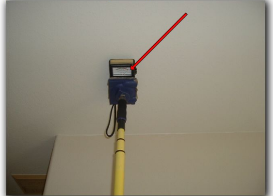
High moisture was detected in ceiling above entry area of the master bathroom linen closet There are cracked tiles at the front entry
