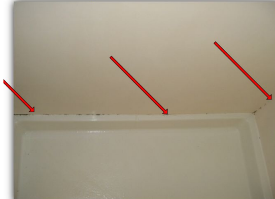
The master shower needs repair to the sealant.
