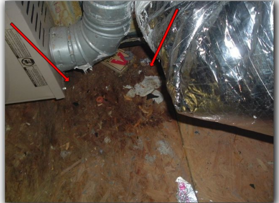
There is evidence of water penetration in the attic at the roof vent.
