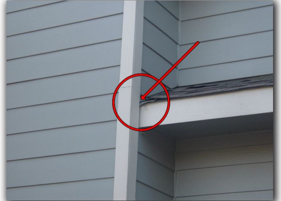
Needs kickout flashing at the front of the house
