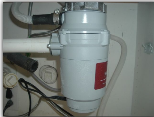
The disposal performed as intended at time of the inspection.
