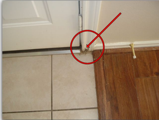
The rear entry door frame and trim has decay.
