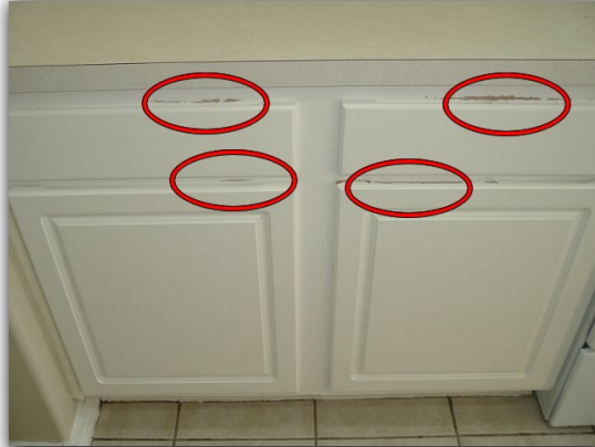
The kitchen cabinets/drawers have visible delamination.
