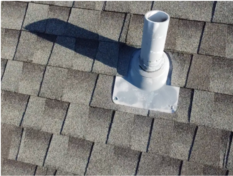
Pipe boot installed using industry best practice. No exposed fasteners.
