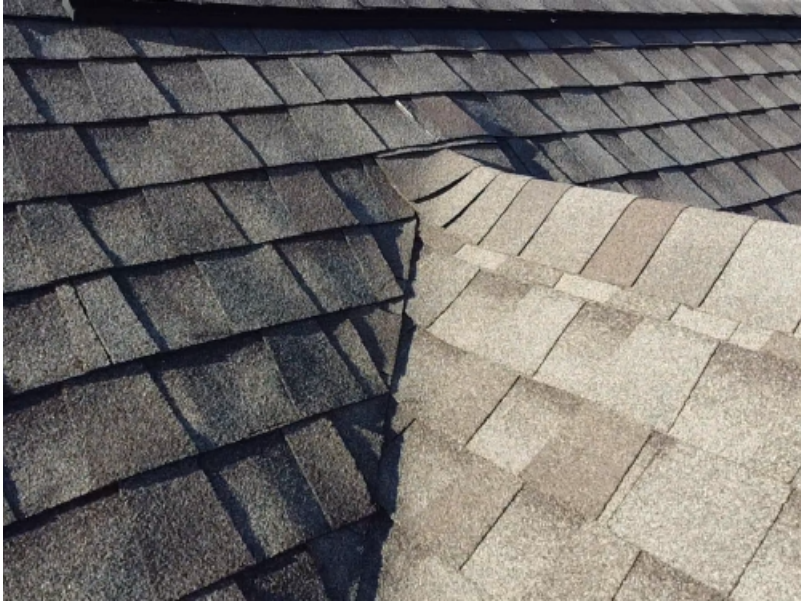
Valley shingles installed correctly
