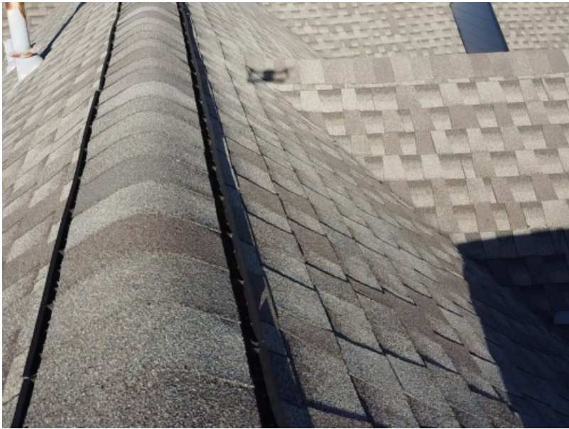
Ridge cap and vent are present and installed properly
