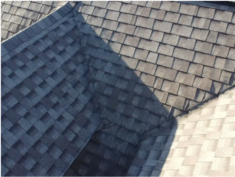
Valley shingles installed correctly
