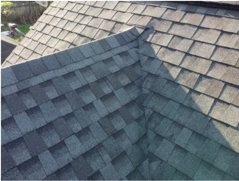
Valley shingles installed correctly
