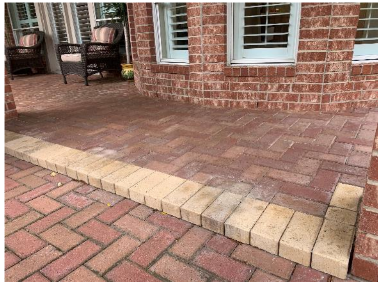
Tile/Pavers obstructing view of the foundation
