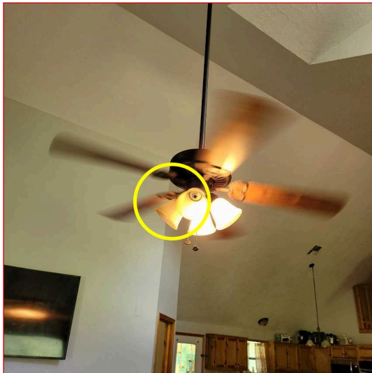
One or more lights not working around the home. Could be burnt out light bulbs.
