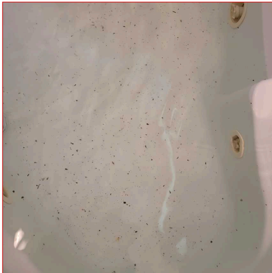
Unit had not been operated in a while. Debris came out of jets.
