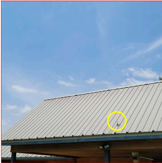
Vent pipes should be painted to protect them from UV rays.
