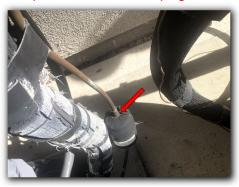
Evidence of past condensation was found on the exterior of the evaporator coil housing(s) of Unit 1 & 3 in the attic. This has lead to moisture related problems, i.e. mildew, rust & corrosion, etc. Recommend further evaluation by a licensed HVAC contractor to determine the needed repairs to correct this problem.
