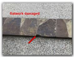
Damaged and missing sealant was found at several areas between the pool coping and decking. All damaged and missing sealant should be repaired/replaced to prevent the leakage of water into these voids.
