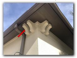
Evidence of previous repairs were found on the exterior of the structure as evident by patching and other signs.
