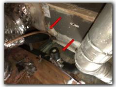
During the inspection of the exterior and interior units of unit 2, labels were found that indicate that refrigerant gases could have been mixed, i.e. R-22 and R-410a. This is typically not allowed and can lead to future problems. We recommend that a licensed HVAC contractor to further evaluate the system to determine if gases have been mixed and if repairs are needed.
