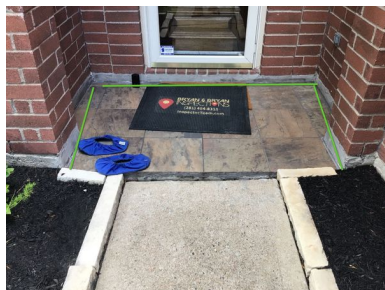
Front, concrete dressing
