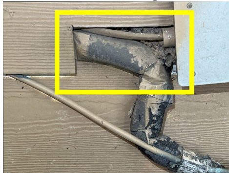
Caulk and seal exterior penetrations
