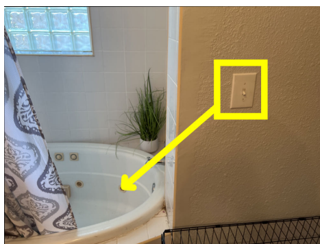
Switch can be operated from bathtub
