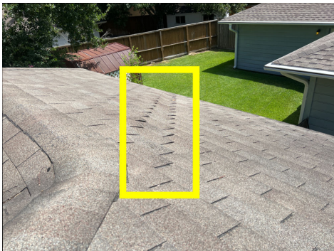
Ridges on roof plane
