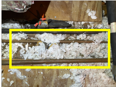
Insulate attic waterlines
