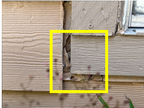
Caulk and seal exterior penetrations
