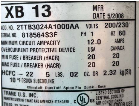
Condensing Unit: 2008 Trane 2 Ton
