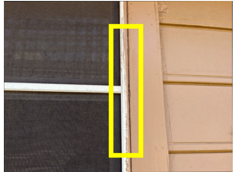
Caulk and seal windows
