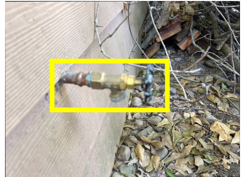
Insulate exterior waterlines
