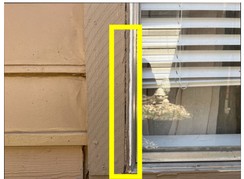
Caulk and seal windows
