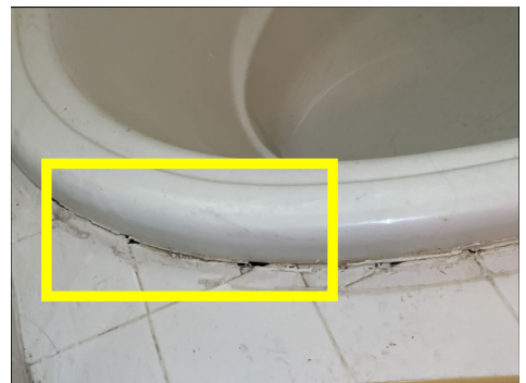
Caulk and seal bathtub
