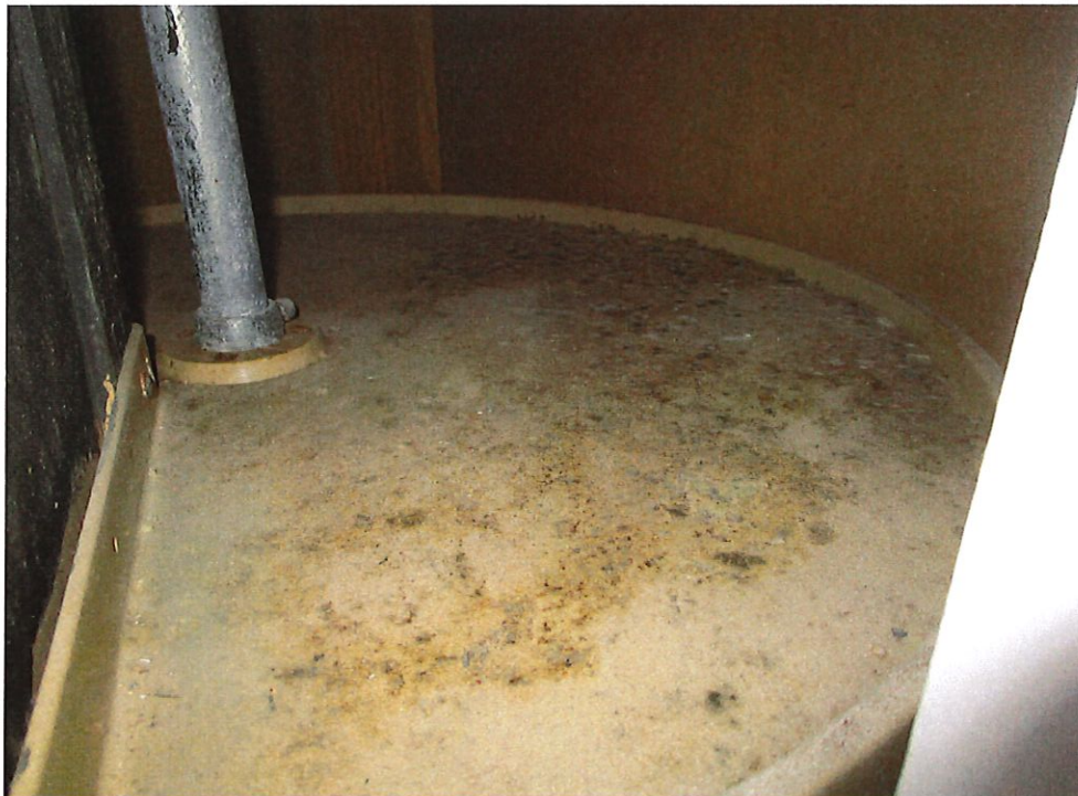
Photo 4 - Mold growth and moisture damage on cabinets and in drawers throughout kitchen.
