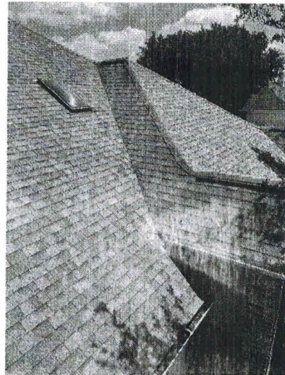
Picture of roof
