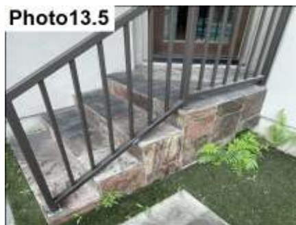
Stair construction is CMU. Seal all terminations.
