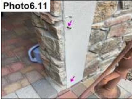
Fastener holes lack sealants.
