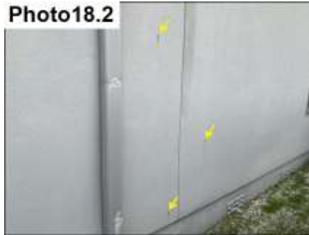
Rust aggregates are present.
