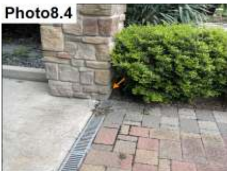
Column base is concrete construction.
