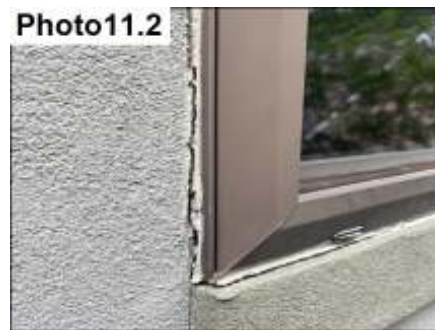
Sealant separation is noted around window frames.
