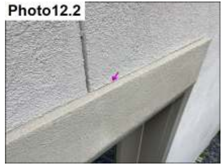
Tops of accent bands lack adequate sealants.
