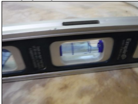
IMPORTANT NOTICE: The flooring in the bathroom was out of level in multiple areas.
