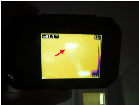
Insulation opportunities in attic
