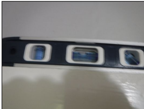
IMPORTANT NOTICE: One or more door frames was noted to be out of level. Further evaluation as to the cause is recommended.
