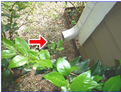
B. Item 1 (Picture) Missing splash blocks B. Item 2 (Picture) Example blocks
