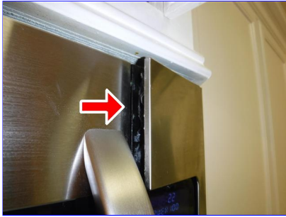
E. Item 1 (Picture) Damaged front housing
