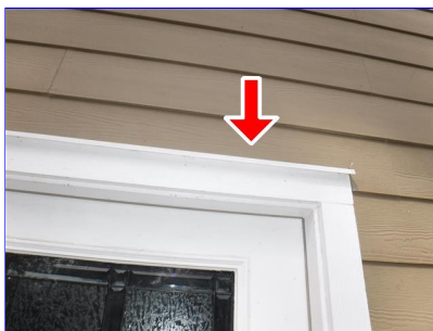
G. Item 2 (Picture) Flashing installed over exterior doors
