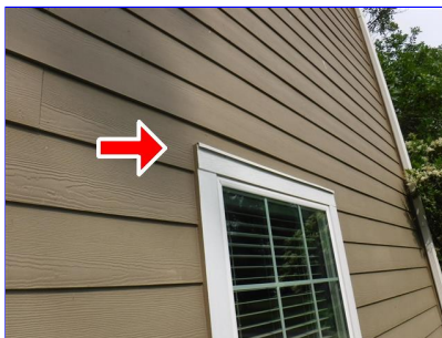
H. Item 2 (Picture) Flashing installed over windows
