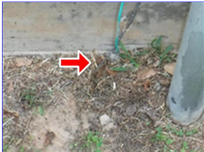
A. Item 3 (Picture) Ground rod present
