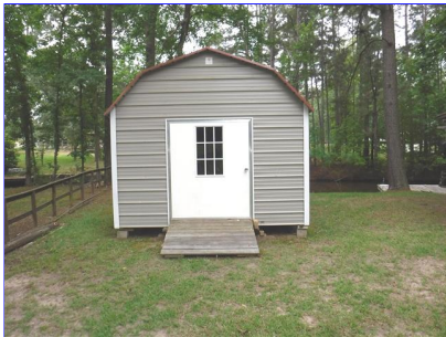
C. Item 1 (Picture) Small wood frame storage building
