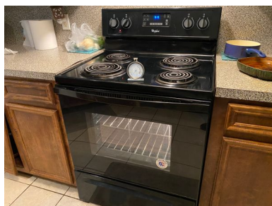
Both units missing anti-tip bracket
