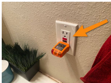
1st Floor Hall Bathroom, unit A
