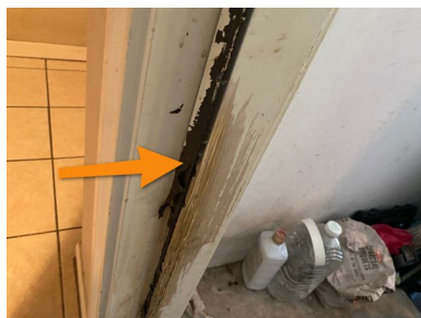
Unit A Garage
