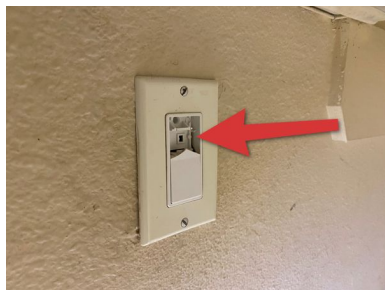
Cover plates were missing at various locations within both units
