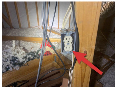
Cover plates were missing at various locations within both units
