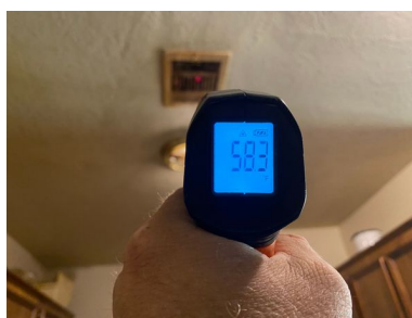
Unit B supply, 12° differential
