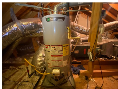
Unit A, attic
