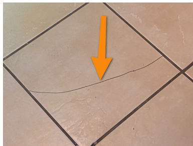
Floor cracks at several locations
