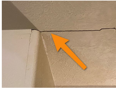
Ceiling cracks
