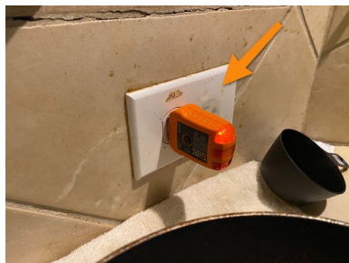
Ungrounded receptacle at one or more locations
