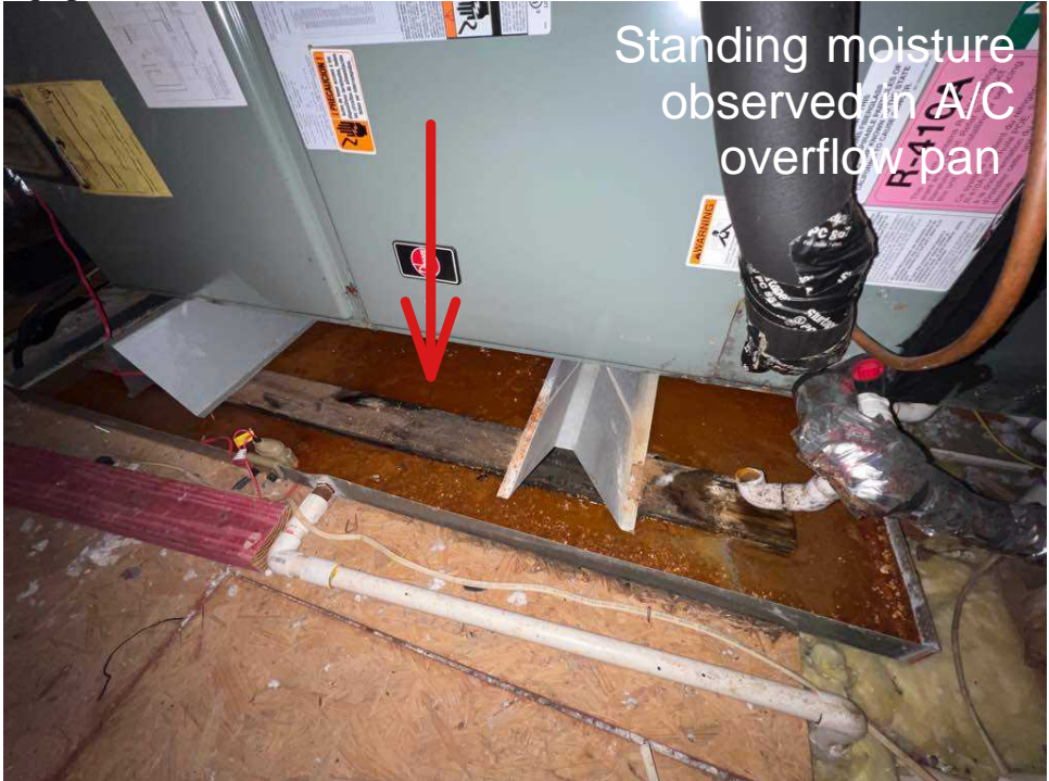
Rust observed in A/C overflow pan (Unit A)
