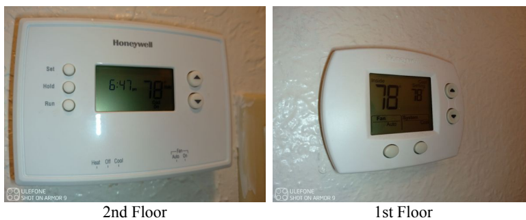
General Infrared Photos of HVAC Equipment:
