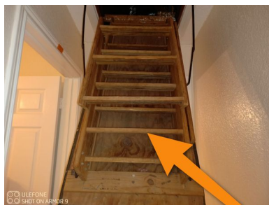
Missing Insulation
