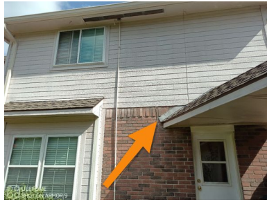
Kickouts Missing
