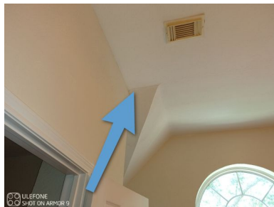
2nd Floor front Left Bedroom
