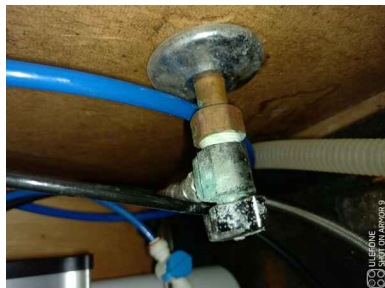
Type of Supply Piping Material: Copper
