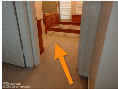
2nd Floor front left Bedroom
