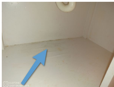
2nd Floor rear Bathroom
