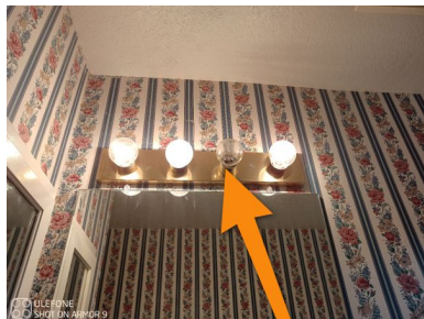
2nd Floor Hall Bathroom
