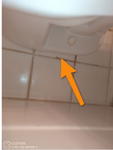
2nd Floor Hall Bathroom
