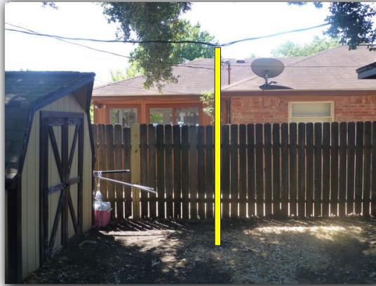
Electrical service wire obstructed by or contacting trees or vines.
