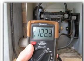
50amp sub-panel-50amp main- 110/220v copper wired breaker service. Breaker wiring, buss bar shields and breakers showed no indications of over heating or arcing and were observed to be in good condition at this time.
