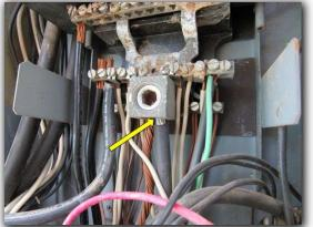
☐ Recommend replacing the pointed fasteners in the service panel dead front with blunt nose fasteners suitable for use with service panels.
