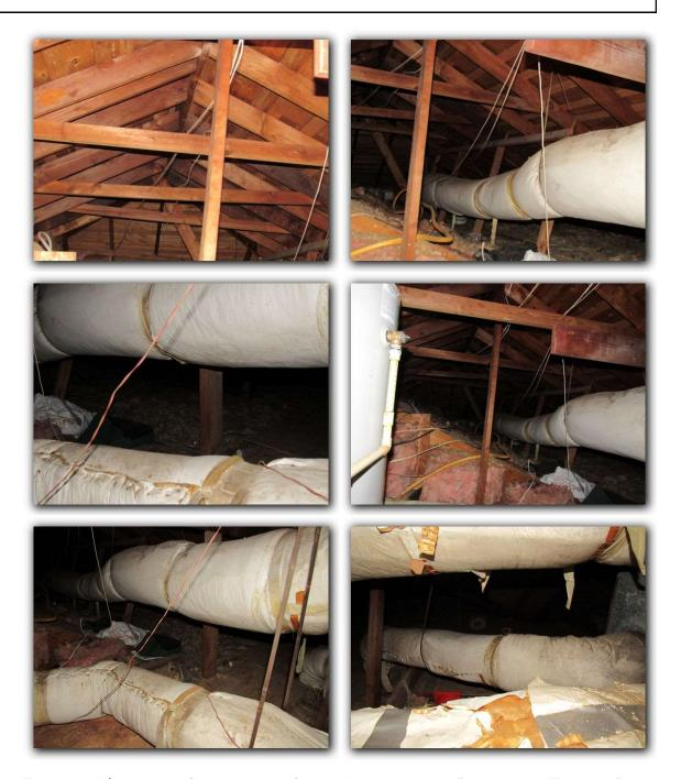
The accessible portions of the attic area of the residence was visually inspected. The overall condition of the visible interior rafters, framing, supports and radiant barrier lined decking appear sound at this time. Insulation in the attic area was observed at a depth of approx. 6-8". Attic ventilation was observed to be continuous soffit vents at the eaves with ridge vents at the ridge. Attic ventilation appears to be adequate at this time.
