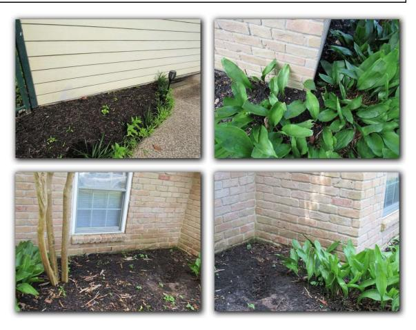
$\square$  It is recommended to make grading improvements along the perimeter of the foundation, as needed, to expose 3-5" of the foundation wall and provide proper drainage away from the foundation.
