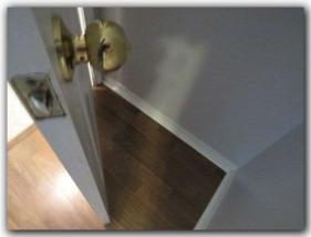
☐ Recommend replacing the missing strike plate at the northeast bedroom entry door jamb.
