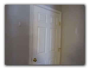
$\Box$  The latch for the east bedroom door improperly installed. Latch observed to be reversed at the time of the inspection.
