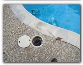
In-ground gunite constructed pool/spa was observed to be structurally sound, no visible cracks in the surfacing or tiling was present at this time. The pool equipment was operated using the timer controller at the equipment area. The 1.5hp-pool pump, 3/4hp booster cleaner pump, cartridge filter system, POLARIS cleaner, returns, skimmers, and spa jets were observed to be operational at the time of the inspection.
