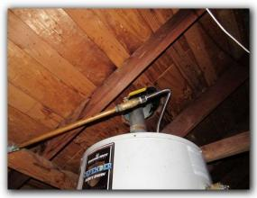
2020 BRADFORD-WHITE 40 gallon gas fired water heater MOD. #RG240S6N, unit was observed to be functional and properly installed at this time. Water temperature was measured at 121 degrees, temperature controls on the water heater can be adjusted for comfort levels.
