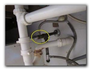
$\square$  Repairs are needed for the leaking valve at the wet bar faucet.
