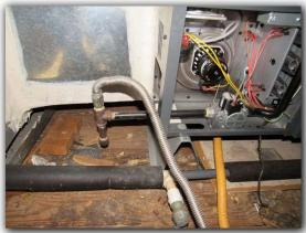
2015 GOODMAN gas fired forced air 60,000 BTU furnace MOD. #GMS80603ANBC. Furnace was operated using the standard manual controls. Furnace operations appeared satisfactory at this time. Burner compartments were relatively free of rust or scale deposits and the flame color was consistent. Furnace installation was also considered satisfactory at this time.
