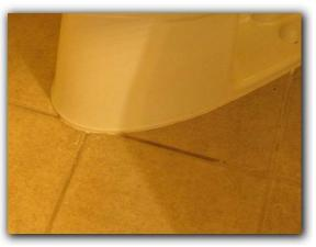
☐ Repairs are needed to secure the loose toilet in the master bath. The toilet should be removed, the closet flange and toilet base cleaned and a new wax ring and closet bolts installed when mounting the toilet.
