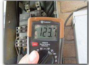
100amp service panel- 110/220v copper wired breaker service. Breaker wiring, buss bar shields and breakers showed no indications of over heating or arcing and were observed to be in good condition at this time.
