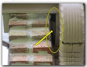
There are small holes in the brick at the right wall near the front corner.
