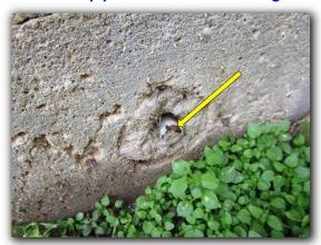
There is exposed aggregate on the right side of the foundation near the front and middle of the right side of the home.
