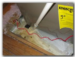
There is evidence of rust on the HVAC casing in the attic.
