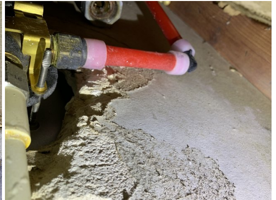
11. Water drops are visible on the hall bathroom tub/shower plumbing lines.
