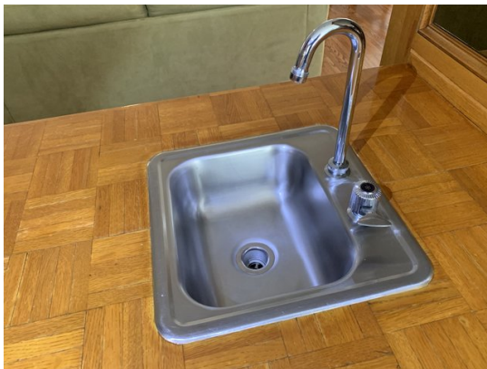
13. The drain for the primary bathroom is operated by rotating the knob by the water over flow. Pushing down on the mechanism can damage the stopper.
