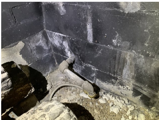
9. The gas valve may need to be secured. The fireplace has a valve that, when opened, will allow the gas to enter into the fireplace. Newer construction would have a valve that opens with a special key, but this house has a door that covers a traditional manual valve. Secure this door so it will be inaccessible to small children.
