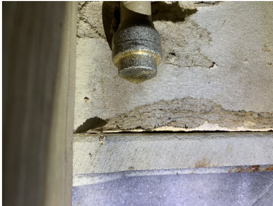
11. Water drops are visible on the hall bathroom tub/shower plumbing lines.
