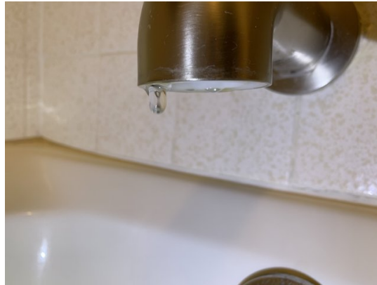
9. The hall bathroom sink hot/cold faucet handles are difficult to operate.
