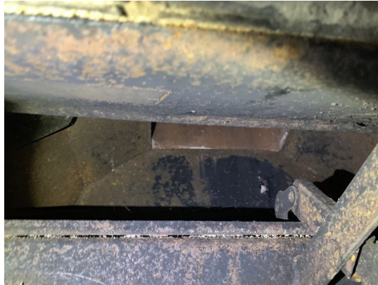
8. The ember screen has separated in one spot.
