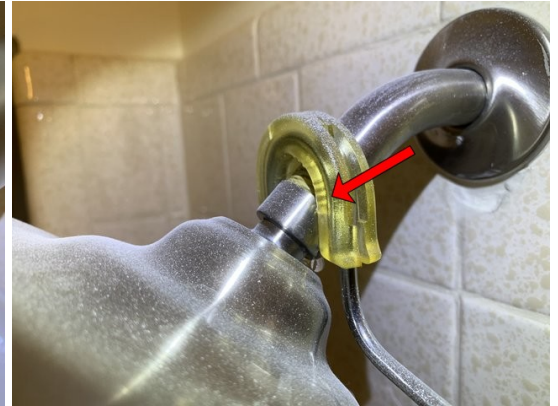
11. Water drops are visible on the hall bathroom tub/shower plumbing lines.
