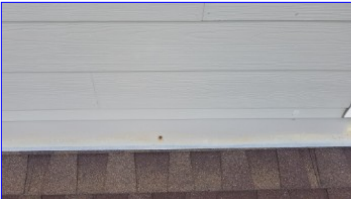
Exposed nails are present on the roofing application. Nailheads should be sealed to prevent leaking and rusty nails should be examined and replaced where needed.
