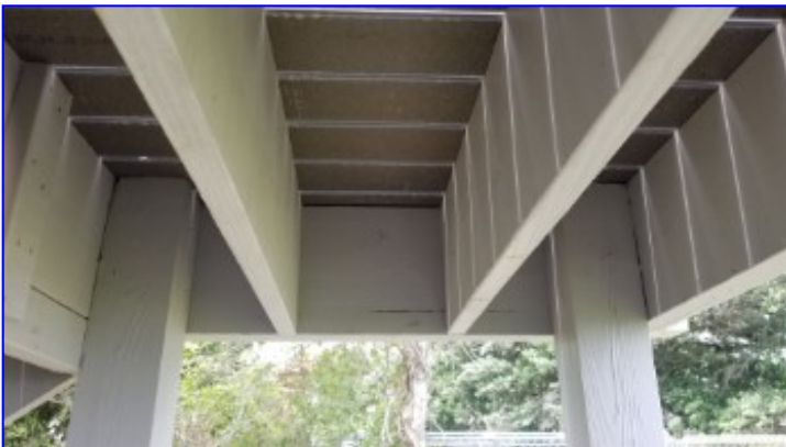
Joist hangers should be installed under the front and rear exterior stair landings to provide proper structural support.
