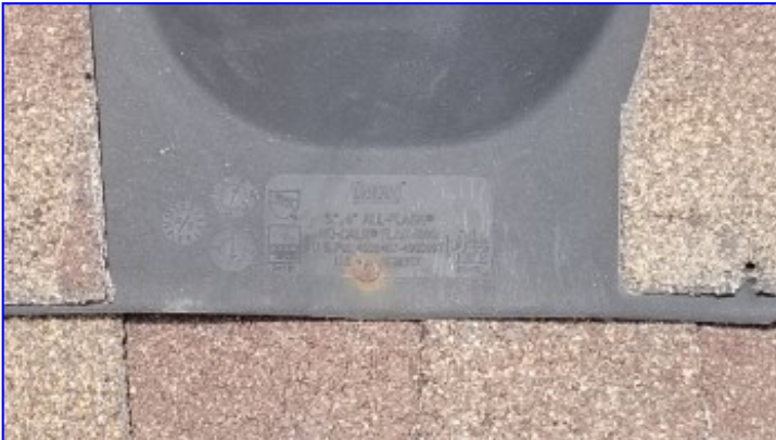
Exposed nails are present on the roofing application. Nailheads should be sealed to prevent leaking and rusty nails should be examined and replaced where needed.
