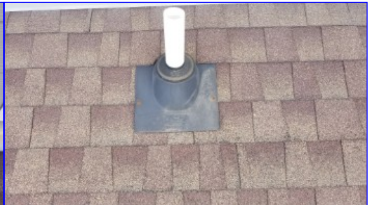
Exposed nails are present on the roofing application. Nailheads should be sealed to prevent leaking and rusty nails should be examined and replaced where needed.
