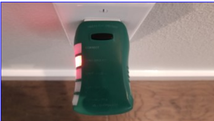
open ground 3rd floor loft
