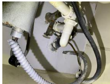
Type of Supply Piping Material: PEX, Galvanized Steel
