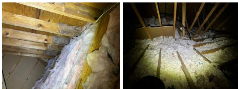
Type of Insulation Material: Blown Fiberglass, Batt Fiberglass
