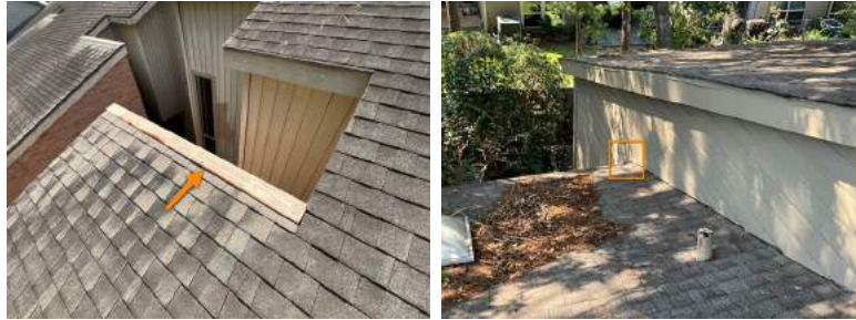
Corroded Flashings
