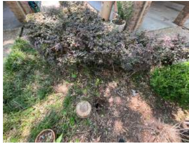
Location of Main Water Supply Valve: Exterior Wall - Left Side
