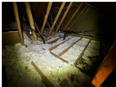
Attic Access Method: Access Hatch/Panel, Knee Wall Access
