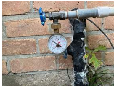
Type of Supply Piping Material: PEX, Galvanized Steel
