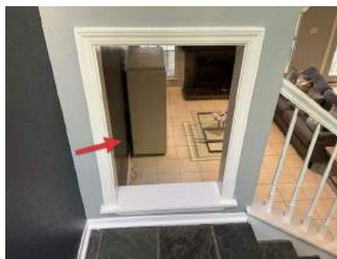
Missing Spindles
