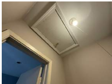
Type of Attic/Roof Ventillation: Ridge Vent
