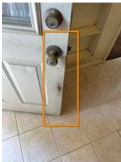
Example Rear Exterior Wall
