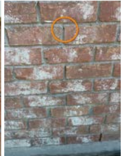
Example right exterior wall
