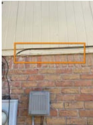
Example right exterior wall
