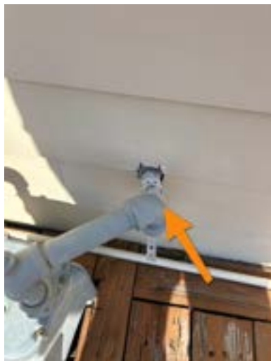
Rear exterior wall
