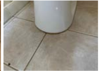
Example laundry room bathroom
