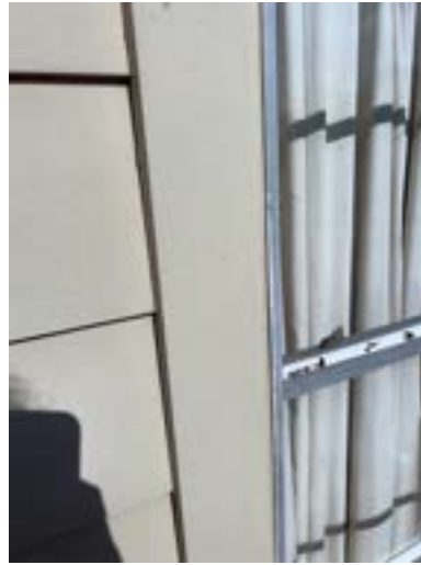
Rear exterior wall
