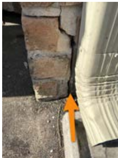
Example left exterior wall
