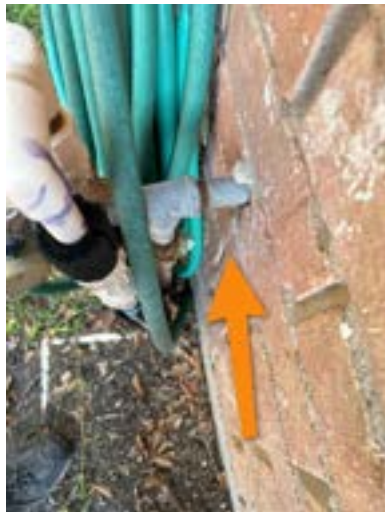
Example right exterior wall
