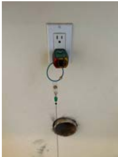
Example, laundry room
