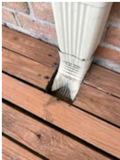
Example rear exterior wall
