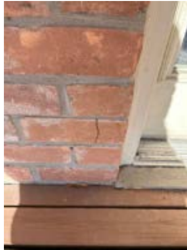
Example rear exterior wall
