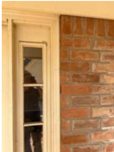
Rear exterior wall
