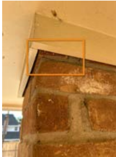
Rear exterior wall
