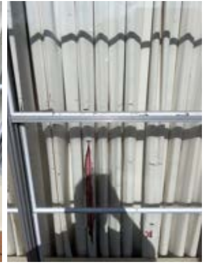
Rear Exterior Wall Example
