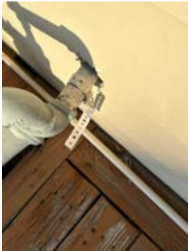
Rear Exterior Wall Example
