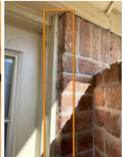
Example rear exterior wall
