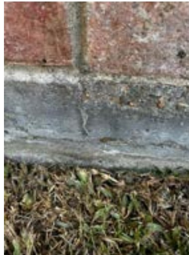
Example right exterior wall
