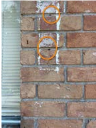
Example right exterior wall
