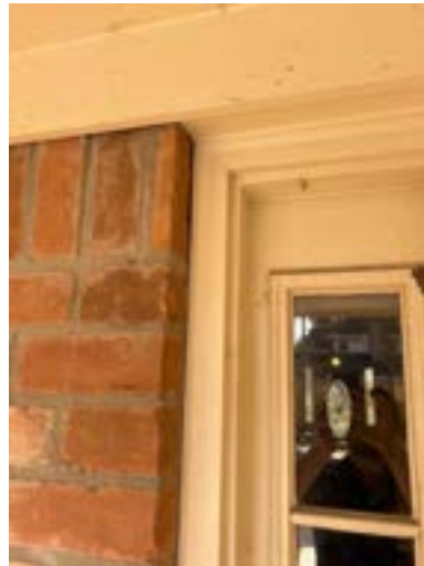
Example rear exterior wall
