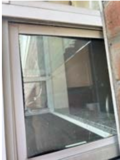
Example left exterior wall
