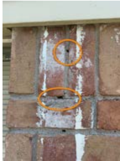
Example right exterior wall
