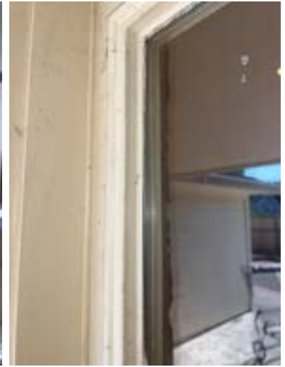
Rear exterior wall
