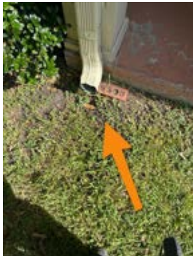
Example Rear Exterior Wall
