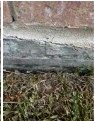
Example right exterior wall
