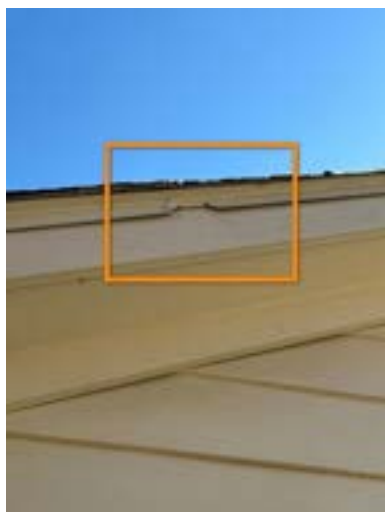
Example guest house right exterior wall
