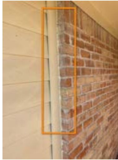
Example Rear Exterior Wall
