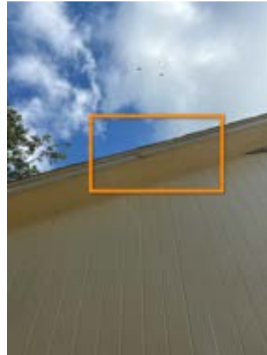
Example Right Exterior Wall
