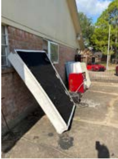
Example left exterior wall
