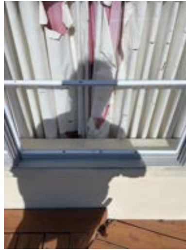
Rear Exterior Wall Example
