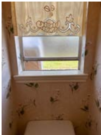
Example, laundry, room window
