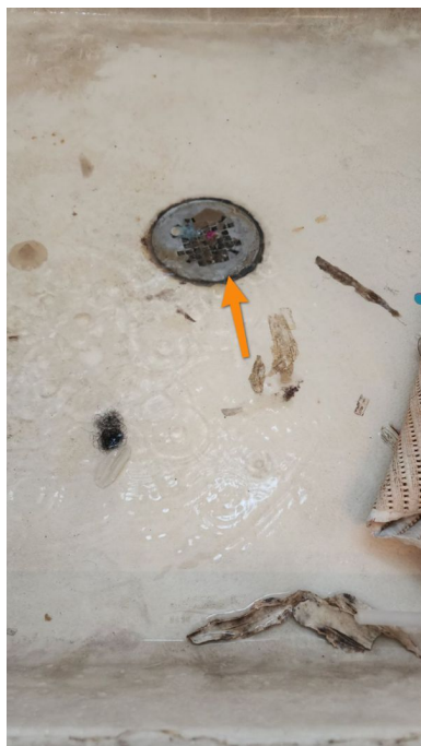
2nd Floor Bathroom shower
