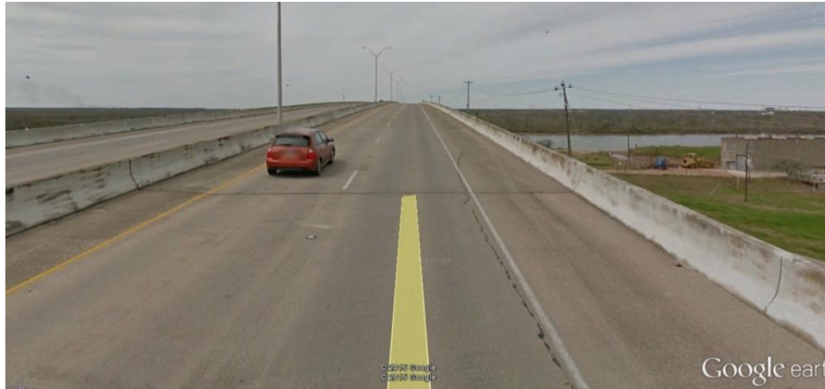
Exhibit 5-3: SH 36 Bridge over the Brazos River
