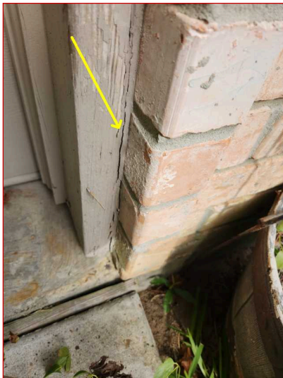
Caulking needed at one or more places around the home/building. This is common maintenance.
