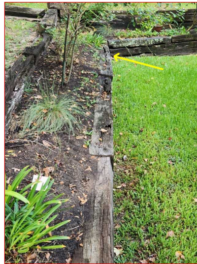
Retaining wall was leaning and is in need of repairs.
