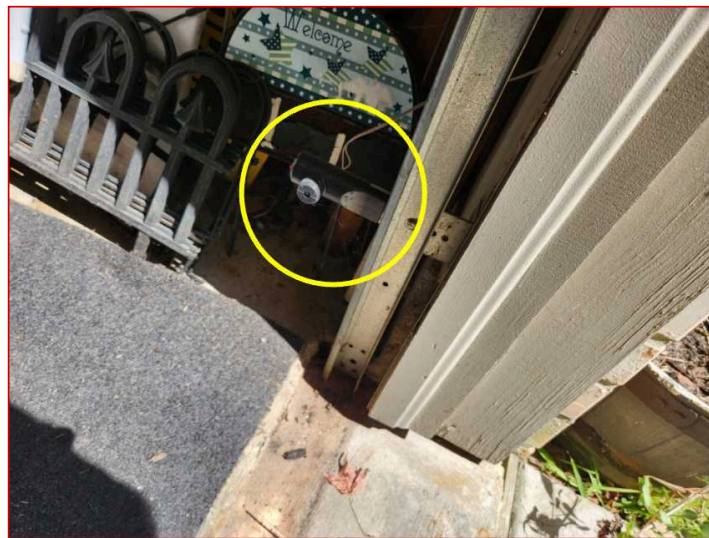
The garage door sensors should be installed within {6"} of the finished floor
