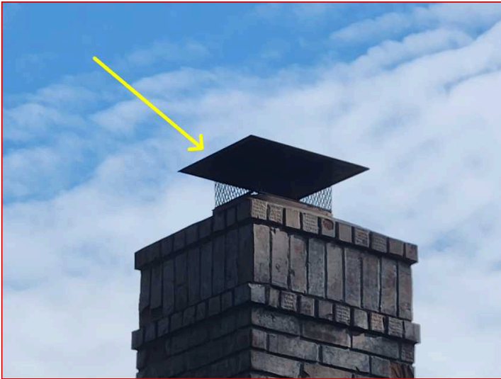
Chimney cap and or rain cap is rusty
