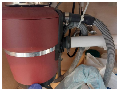
High Drain Loop Backflow Prevention
