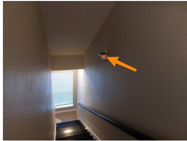
1st Floor Stairway
