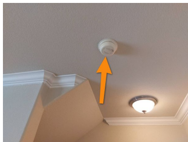
2nd Floor and Several Locations
