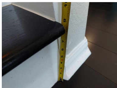
2nd Floor and Several Locations
