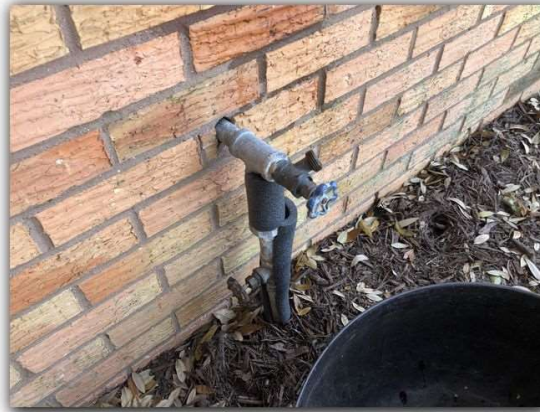
The rear hose bib faucet handle is damaged.
