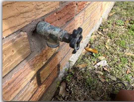
The rear hose bib faucet handle is damaged.
