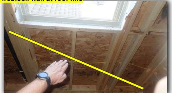
Fireblock wall at roof line
