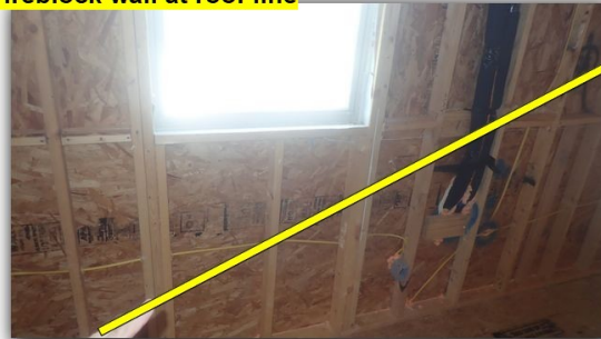
Fireblock wall at roof line
