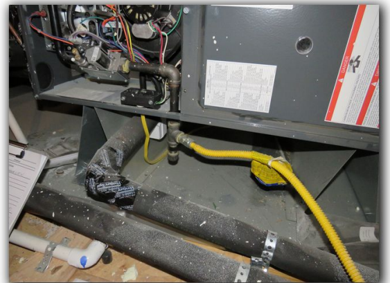
2021 GOODMAN gas fired forced air 40,000 BTU furnace MOD. #GMVC960403BN.
