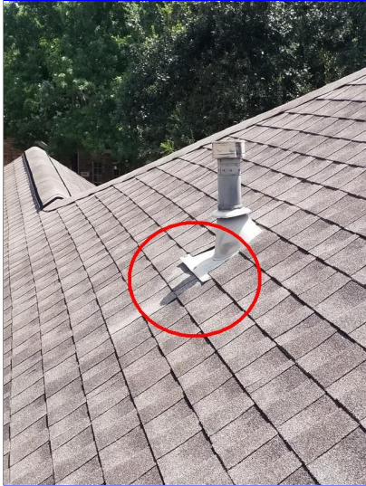
C. Item 1 (Picture) Roof area
