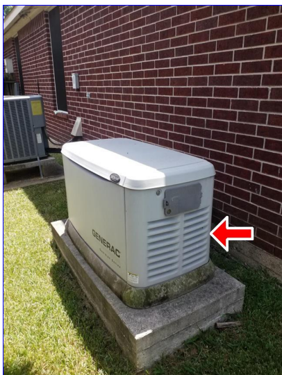
C. Item 1 (Picture) Right side of home
