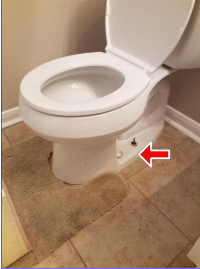
A. Item 1 (Picture) Shared bathroom
