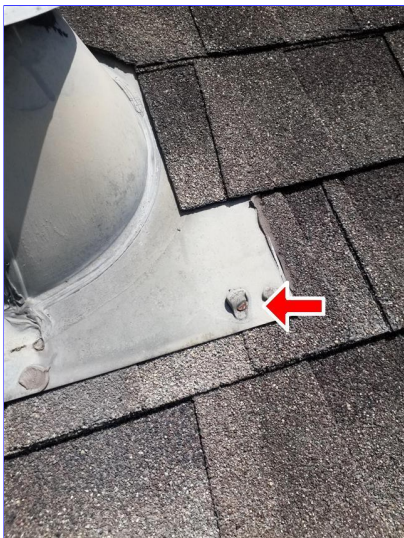
C. Item 2 (Picture) Roof area
