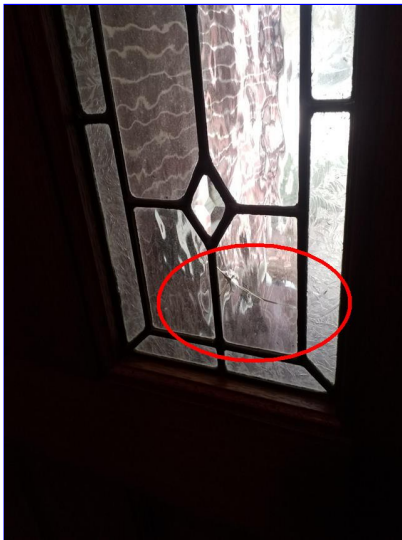
H. Item 1 (Picture) Entry door
