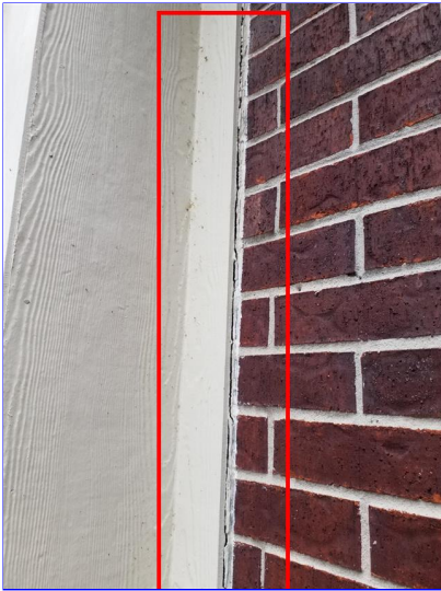
L. Item 2 (Picture) Multiple areas exterior
