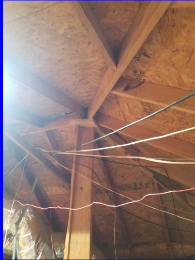
Stick build without radiant barrier
