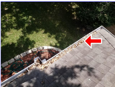
B. Item 3 (Picture) Gutters
