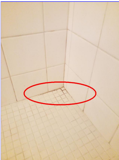
L. Item 4 (Picture) Master bathroom shower stall
