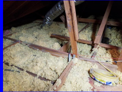
Blown insulation 10 inches
