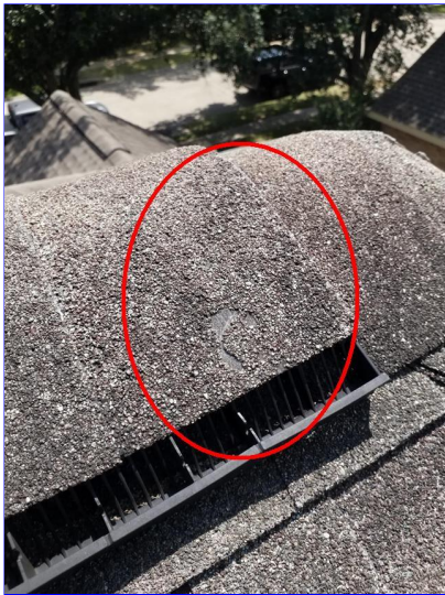
C. Item 3 (Picture) Roof area
