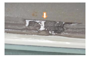
Observed the absence of approved corrosion–resistant flashing above the projecting trim above the window at the
