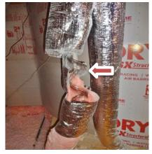
Observed media filters have been incorporated in the HVAC systems and are located adjacent to the return air side
