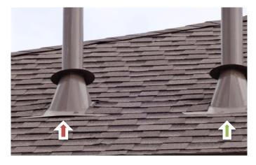
• Observed raised singles at the hips at the rear of the center ridge above the 2<sup>nd</sup> floor. In need of improvement to prevent further / future wind uplift and moisture penetration.
