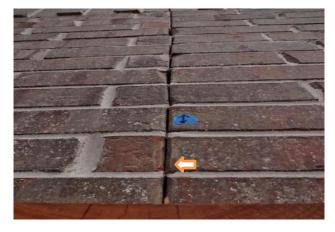
Observed open cavities in the mortar at the lintel and wall area above the left side windows at the study. In need of
