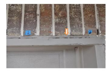
• Observed the absence of weep holes in the stone veneer wall at the right side of the front porch. Under current building standards, weep holes shall be installed in the lower course of the brick veneer, at 33 inch intervals, to help vent and drain moisture from within the wall cavity. In need of improvement.
