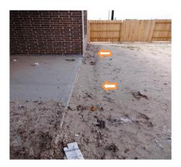
• Observed down spouts serving the gutter system at the front of the house are terminating too close to the foundation causing soil. I recommend installing a splash block under the down spout or a down spout extension that will deposit water at least five feet away from the foundation. Some affected areas have been identified with blue tape and an "X".
