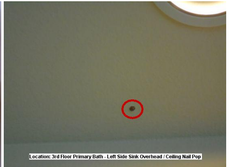
Nail pops in ceiling and in walls in one or more places throughout this home. Mostly these are cosmetic and not serious to be reported. Repair at your leisure.
