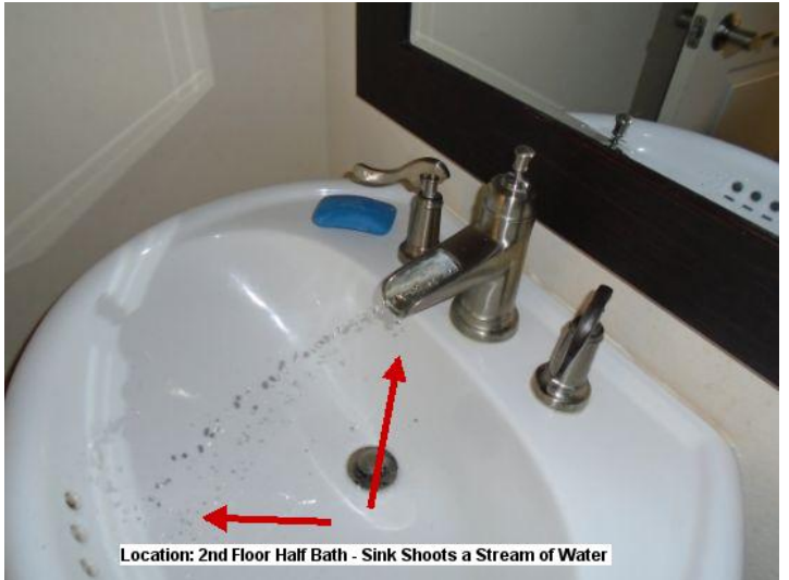
In one or more bathroom sinks, the pressure and angle of water flow exceeds the limits of the sink size.
