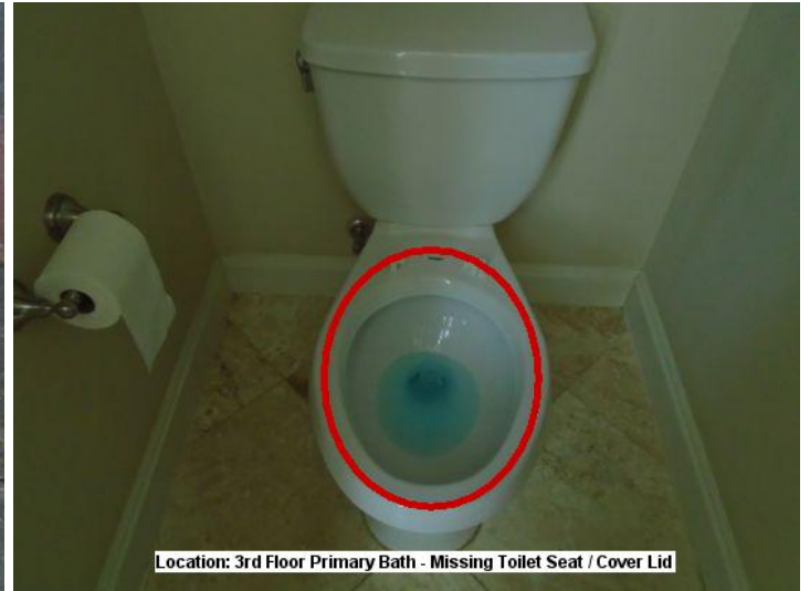
Primary Bathroom toilet seat and lid were missing during today's inspection.
