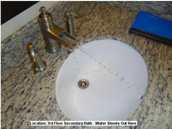
In one or more bathroom sinks, the pressure and angle of water flow exceeds the limits of the sink size.
