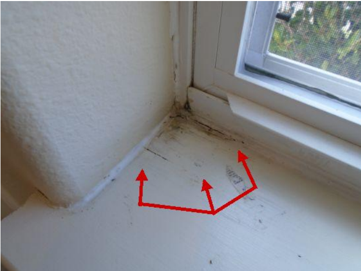
On one or more window sills, evidence of cracking and or paint peeling.
