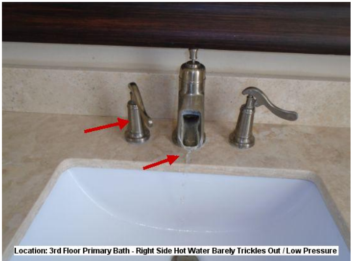
In one or more sinks the flow of water is a trickle even with water turned on all the way.
