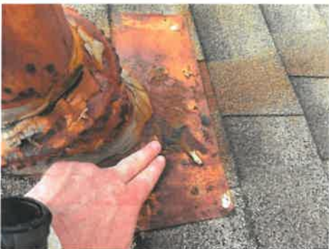
Rusted flashing
