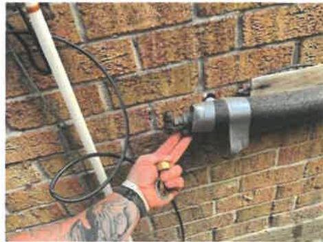
A backflow preventer is recommended
