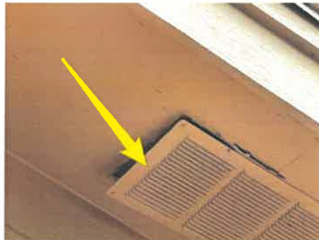
Opening in soffit/ secure soffit vent in place
