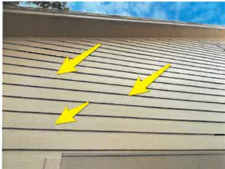
Seal all siding joints
