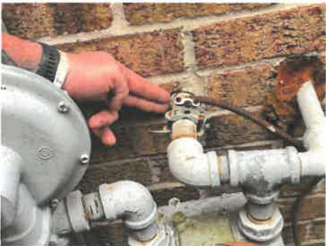
Caulk/seal all exterior wall protrusions
