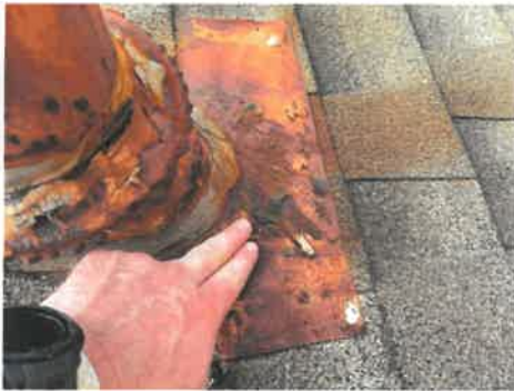
Rusted flashing
