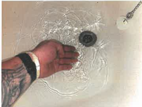
2nd floor hall bathroom: slow drain
