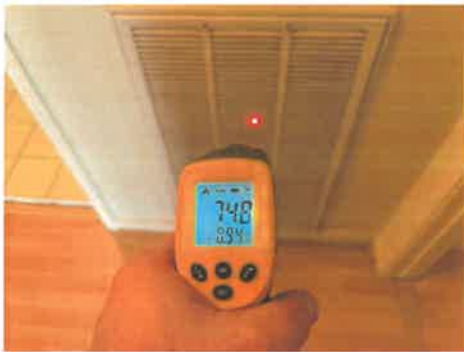
2nd floor return air temperature 74 degrees
