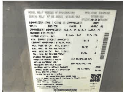
1st floor unit: 2018 model 3 ton unit
