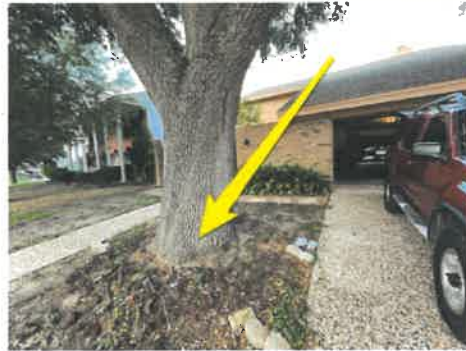
Tree in close proximity of structure
