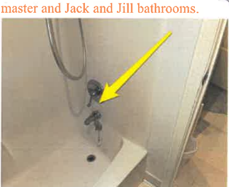
Caulk/seal all shower and tub wall protrusions
