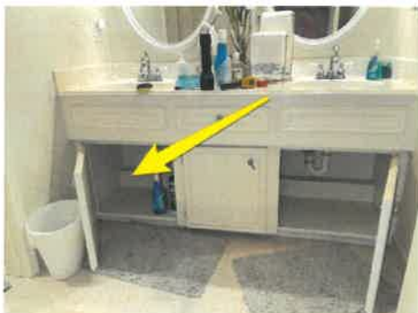
Corrugated drain line present
