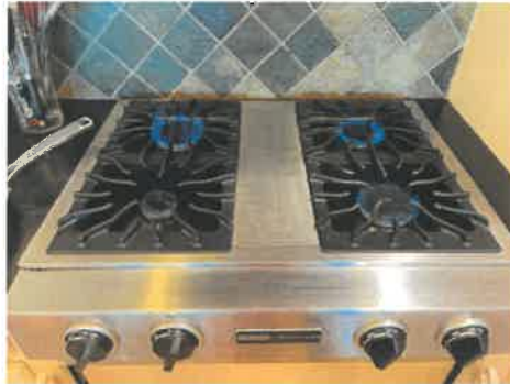
All gas burners on
