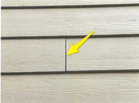
Seal all siding joints
