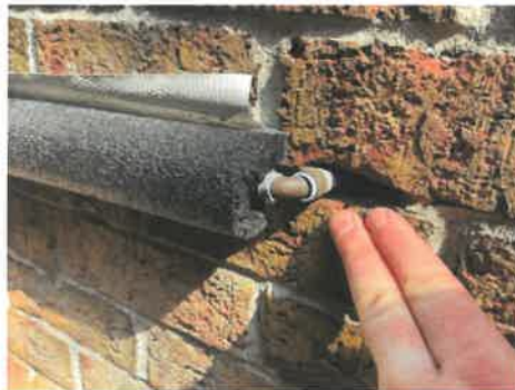
Caulk/seal all exterior wall protrusions
