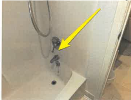
Caulk/seal all shower and tub wall protrusions
