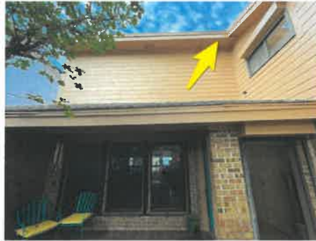
Opening in soffit/ secure soffit vent in place
