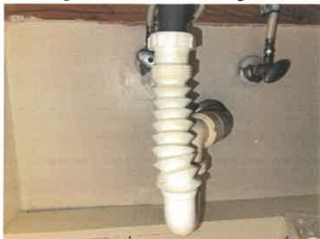
Corrugated drain line present
