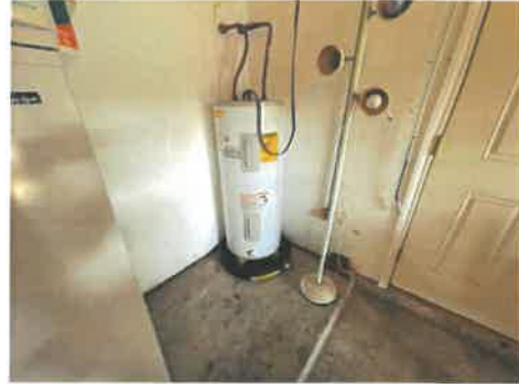
Improper elevation
