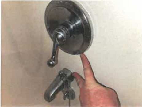
Caulk/seal all shower and tub wall protrusions
