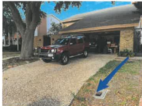
Front: water meter
