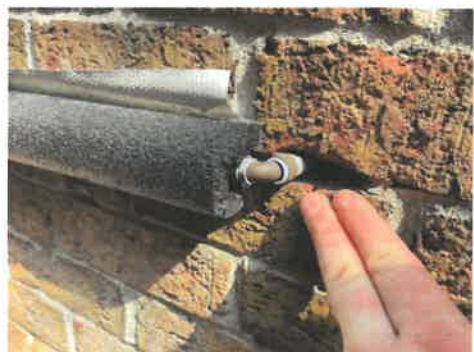
Caulk/seal all exterior wall protrusions
