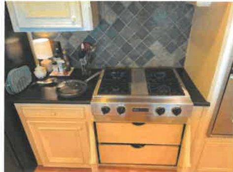
All gas burners on
