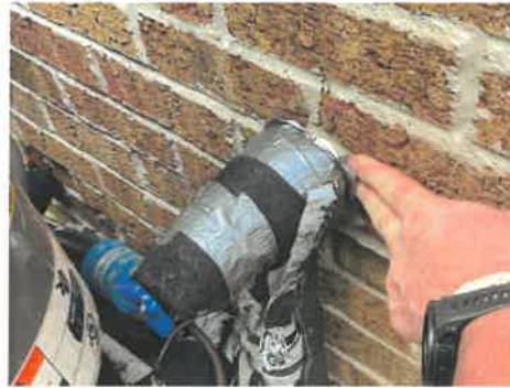
Caulk/seal all exterior wall protrusions
