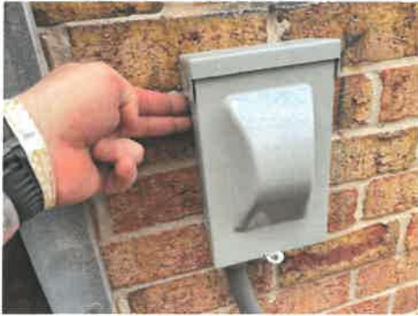
Caulk/seal all exterior wall protrusions
