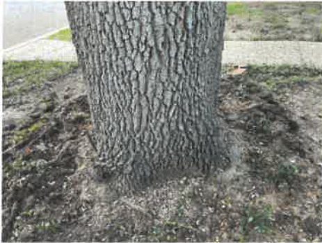
Tree in close proximity of structure
