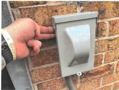
Caulk/seal all exterior wall protrusions
