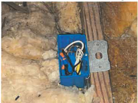
Attic: open junction box
