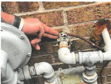
Caulk/seal all exterior wall protrusions
