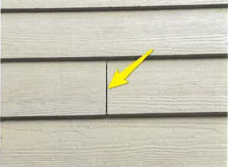
Seal all siding joints
