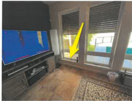
Living room: Window screen damage
