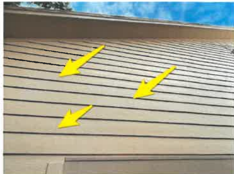
Seal all siding joints
