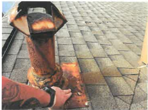
Rusted flashing
