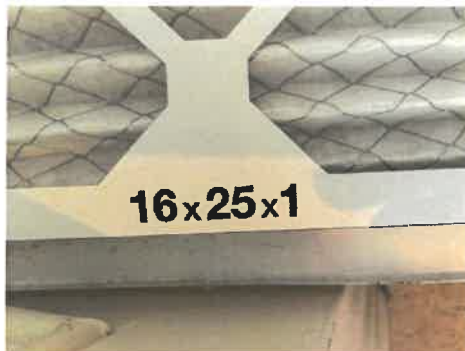
Air filter size 1st floor
