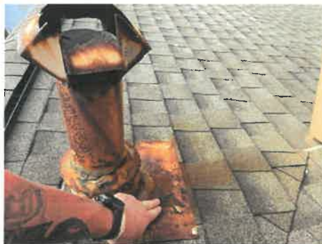
Rusted flashing
