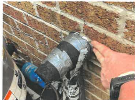
Caulk/seal all exterior wall protrusions
