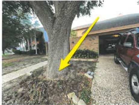
Tree in close proximity of structure
