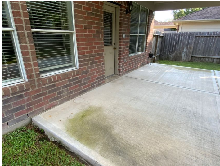
Patio blocking visual inspection of foundation at Back of home.
