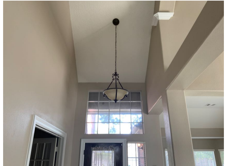
Inoperative light at entryway.
