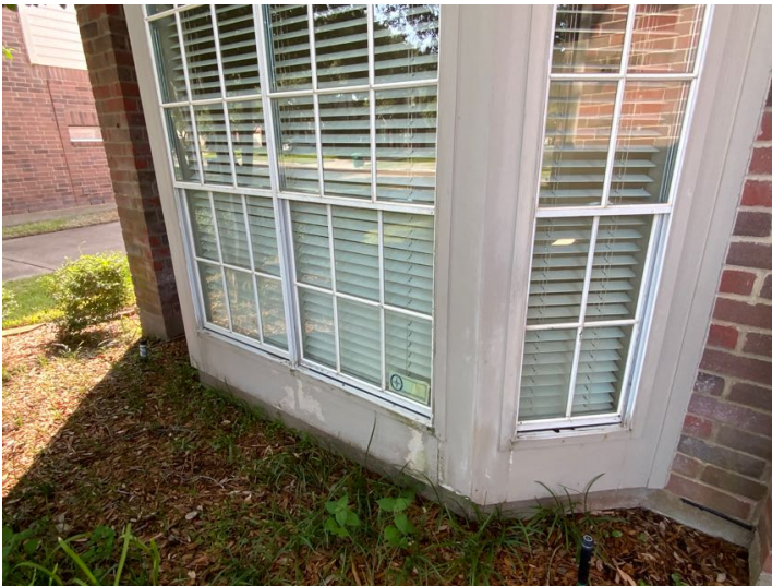
Missing screens throughout home.
