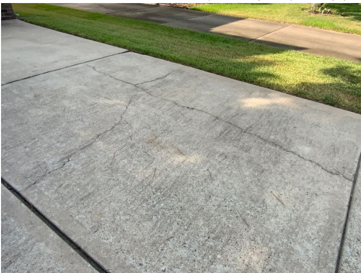
Driveway cracks.
