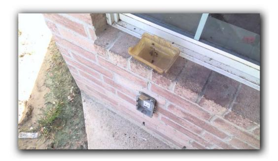
A ground fault circuit interrupter (GFCI) outlet at the exterior of the home did not respond correctly to testing during the inspection. This receptacle should be replaced.
