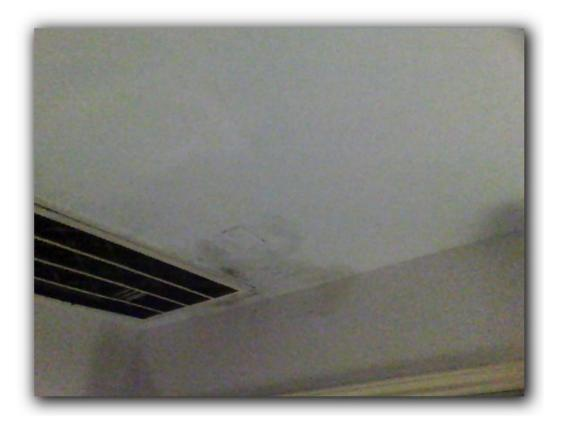
Thermal anomalies were observed in the ceiling of the second floor indicating missing or compressed insulation. Improvements should be made as necessary.
