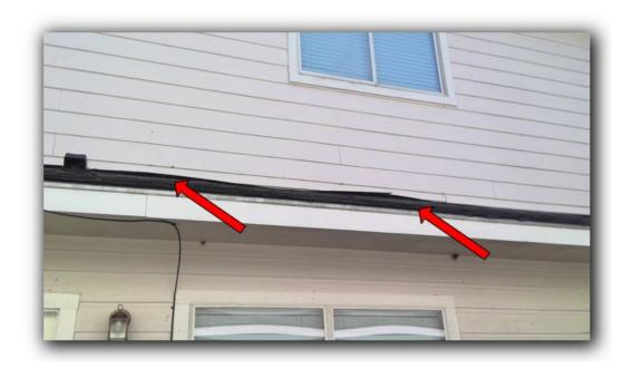
Older roof, approximately 1/2 of serviceable life expectancy. Observed one or more of the following conditions: brittle, cracked, curled ends, and/or excessive granular loss of shingles.
