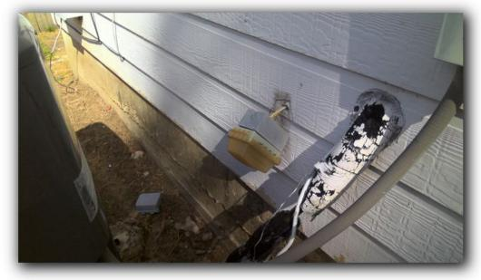
The weather cap on the exterior outlet is damaged and should be replaced.
