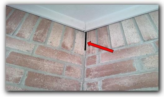
Minor cracks were noted on interior walls at the exterior of the home. This condition is mainly cosmetic in nature and should be patched.
