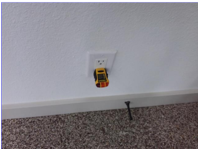
B. Item 16(Picture) master bedroom
