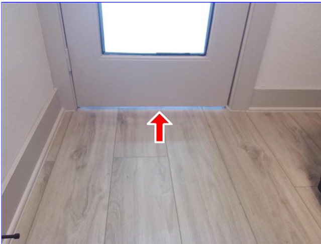
G. Item 1(Picture) laundry room
