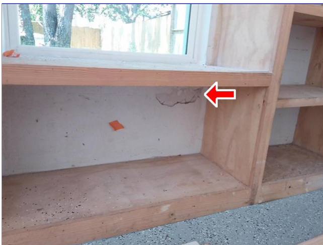
E. Item 5(Picture) garage
