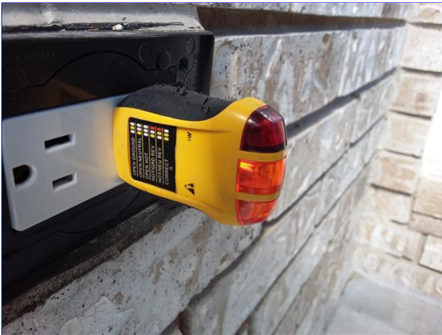
B. Item 11(Picture) main entry exterior
