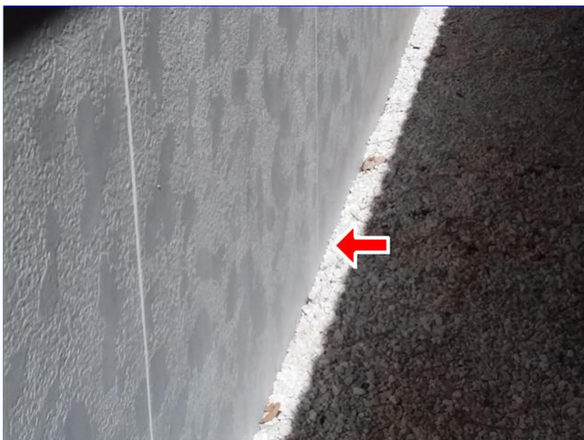
E. Item 1(Picture) garage exterior
