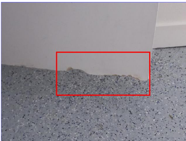
G. Item 4(Picture) garage storage door
