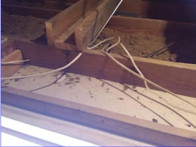
B. Item 10(Picture) garage attic
