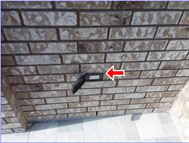
B. Item 6(Picture) main entry exterior
