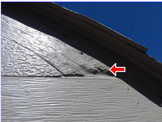
E. Item 3(Picture) front left
