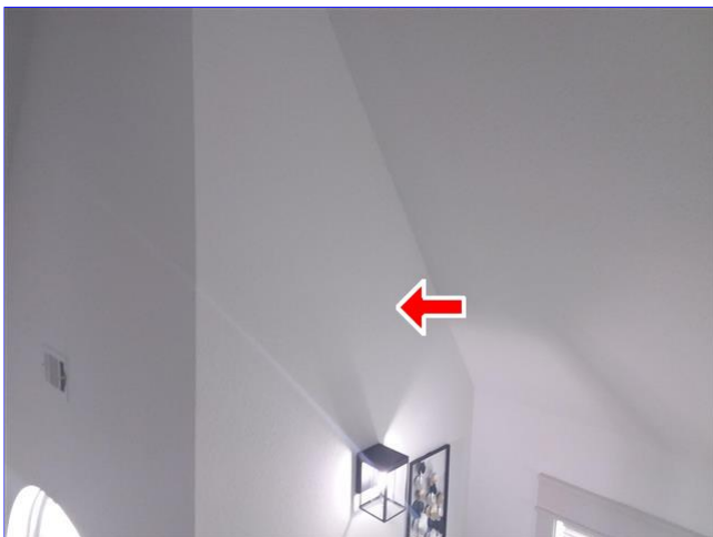
D. Item 8(Picture) stairway
