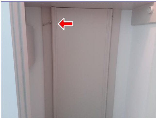
G. Item 3(Picture) storage under stairs
