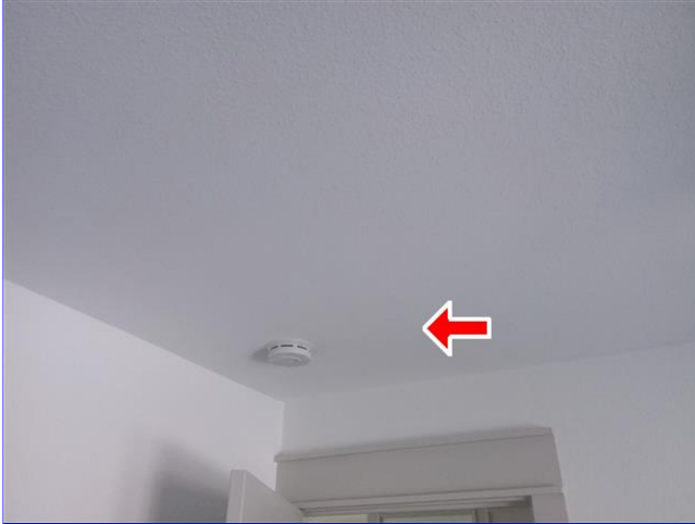
D. Item 6(Picture) right upstairs bedroom
