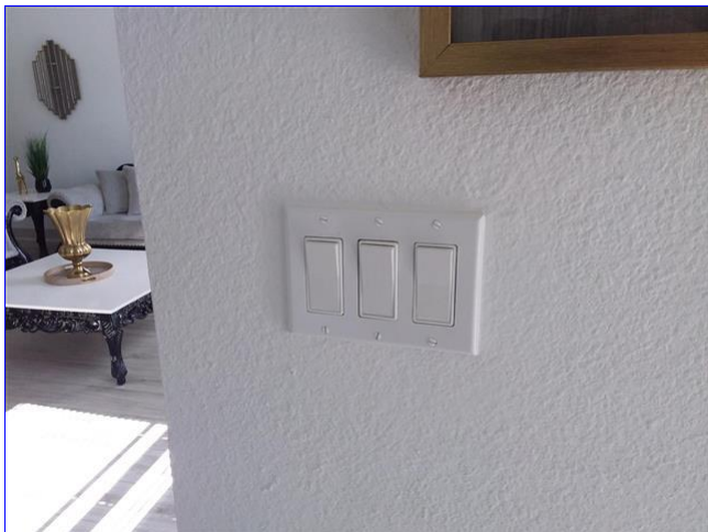
B. Item 14(Picture) living room
