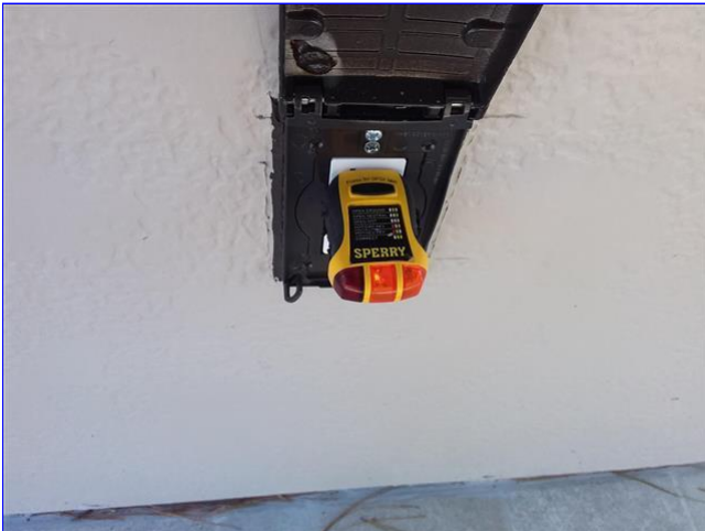
B. Item 12(Picture) upper balcony
