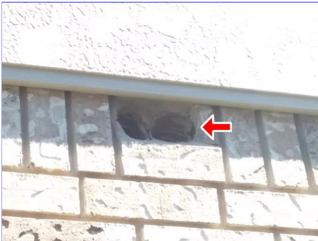
F. Item 1(Picture) left exterior
