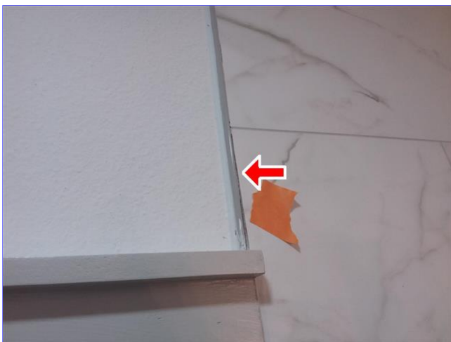
E. Item 4(Picture) master bathroom
