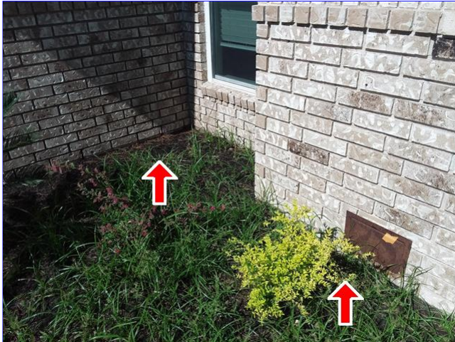
B. Item 1(Picture) front of home
