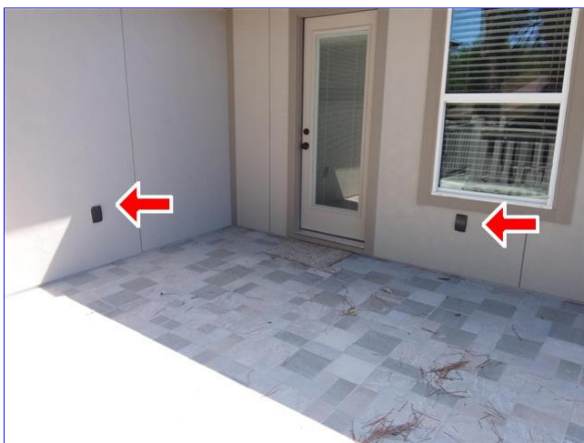
B. Item 4(Picture) upper balcony cannot be opened
