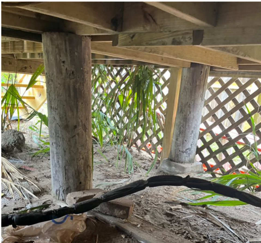
Figure 12&13: 8'x8' laundry/kitchen area contains no beams and toenailed joists. Replace with joist supported with a beam on each end of joists. Replace random wooden post with cinder block piers resting on a concrete pier pads
