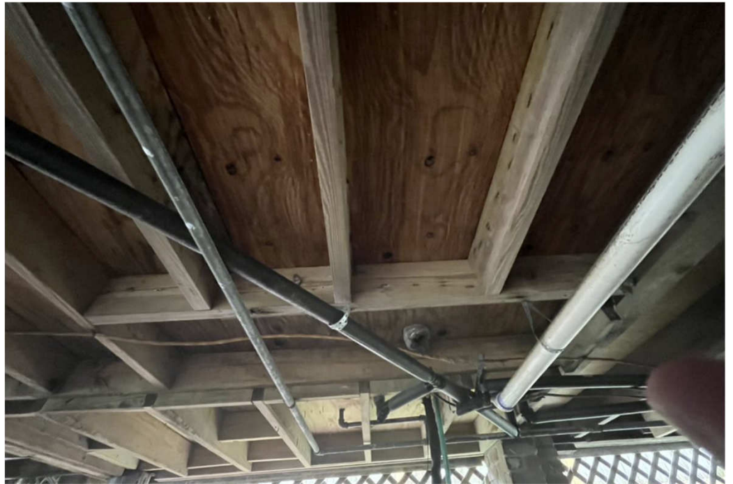
Figure 12&13: 8'x8' laundry/kitchen area contains no beams and toenailed joists. Replace with joist supported with a beam on each end of joists. Replace random wooden post with cinder block piers resting on a concrete pier pads
