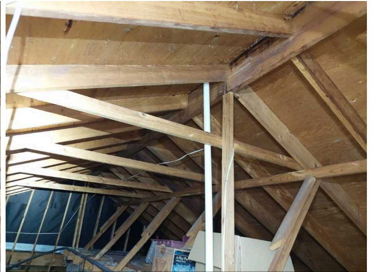
Picture of attic space
