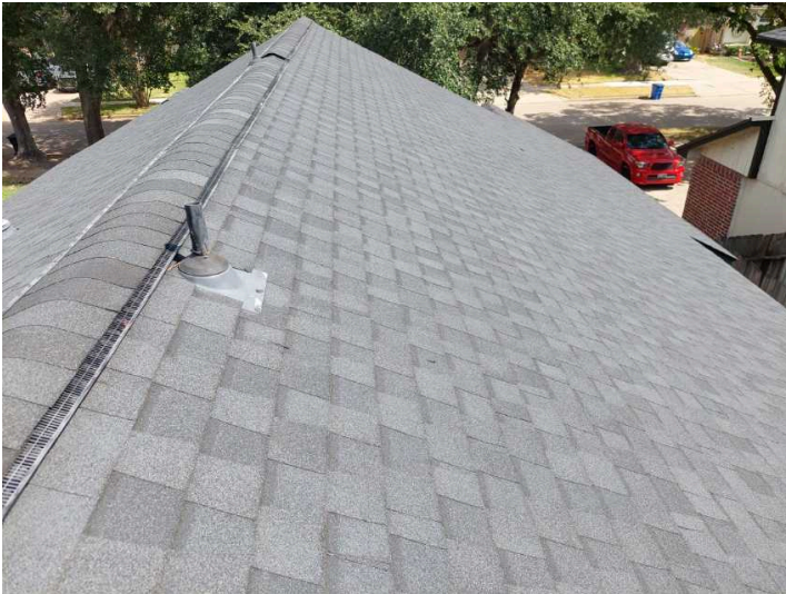
Picture of roof
