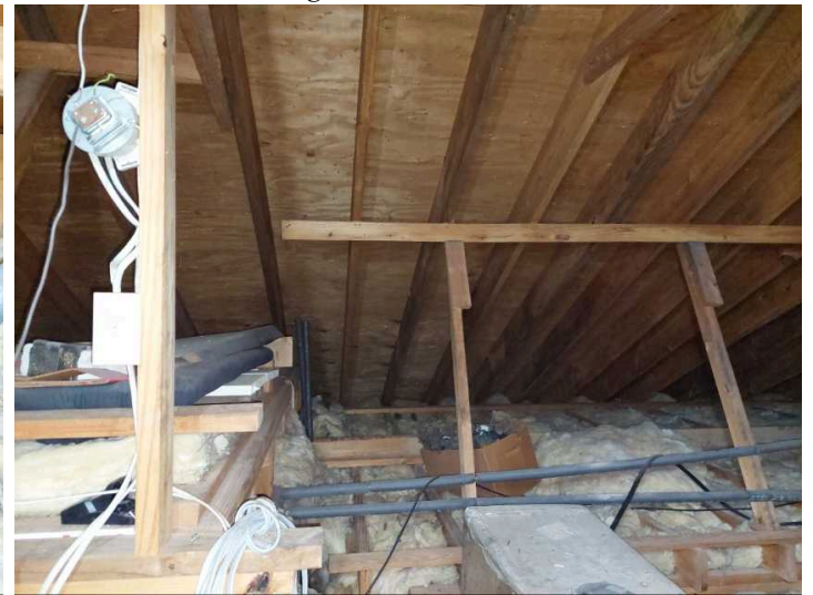
Picture of attic space
