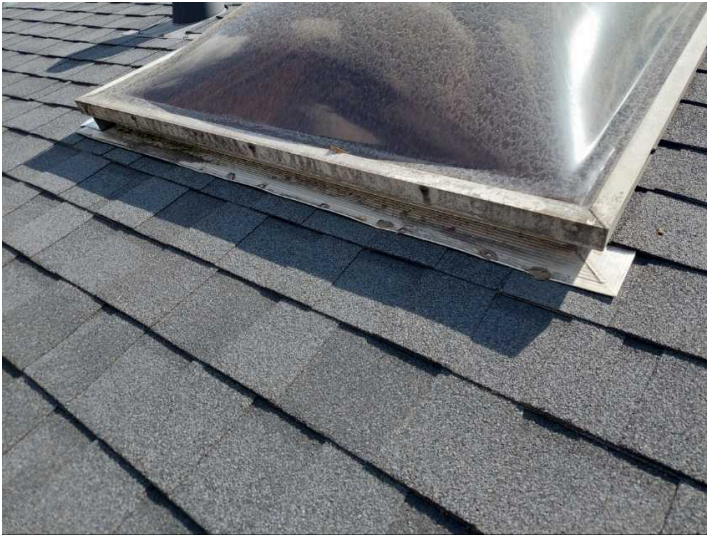
Picture of roof
