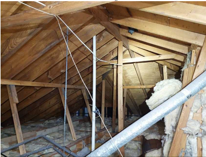
Picture of attic space
