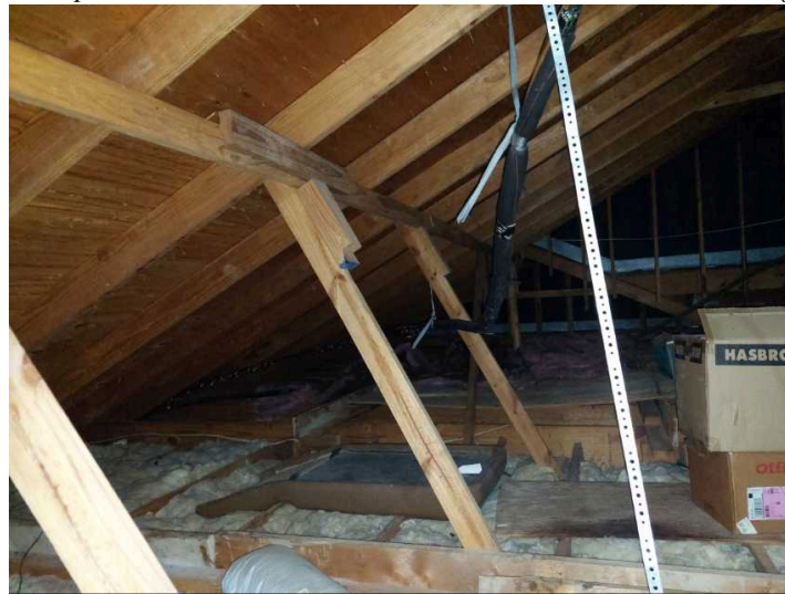
Picture of attic space
