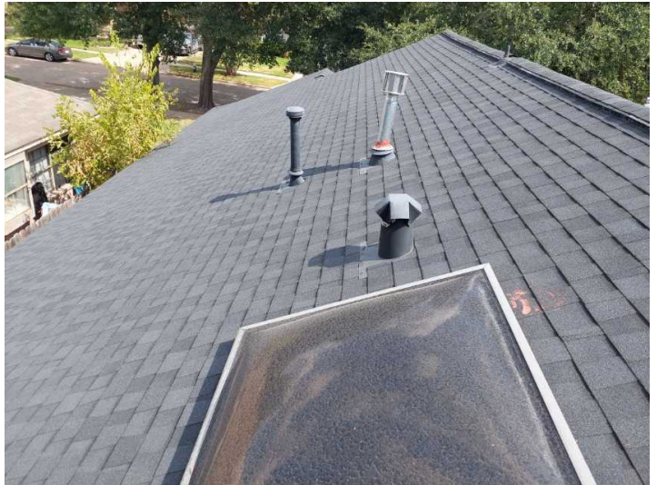
Picture of roof
