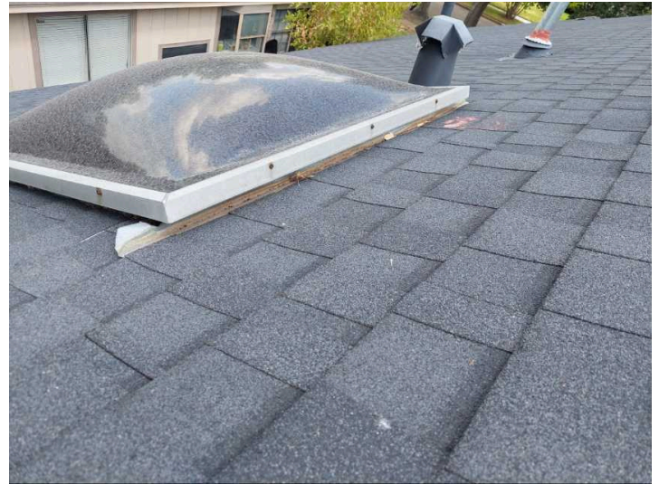
Picture of roof
