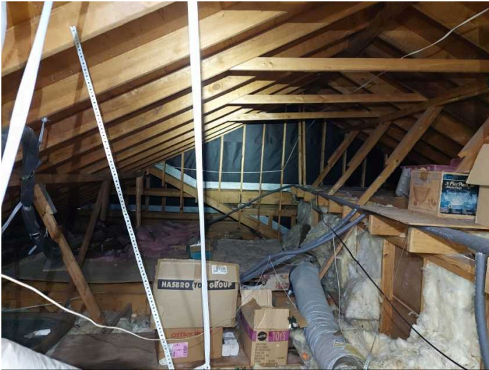
Picture of attic space
