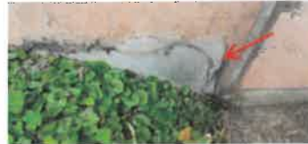
A plastic cover is present on rear exterior wall near porch.
