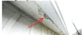
Discoloration on soffit present along back left corner of home.
