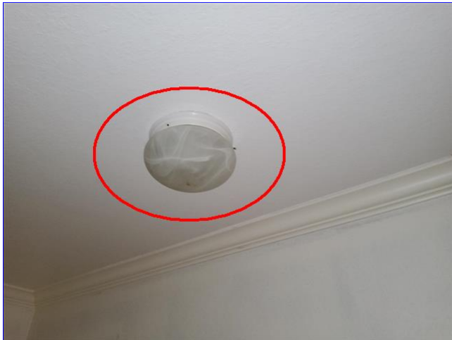
B. Item 8 (Picture) Hallway area
