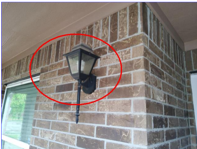
B. Item 9 (Picture) Front porch area
