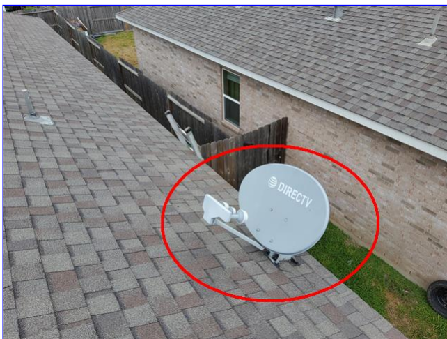
C. Item 2 (Picture) Roof
