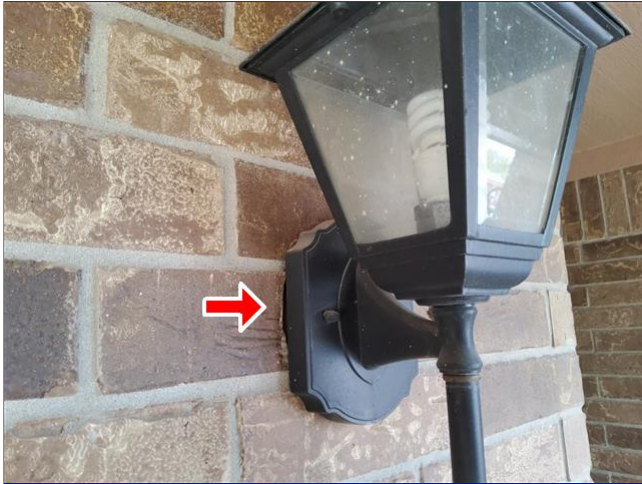
E. Item 1 (Picture) Front porch area
