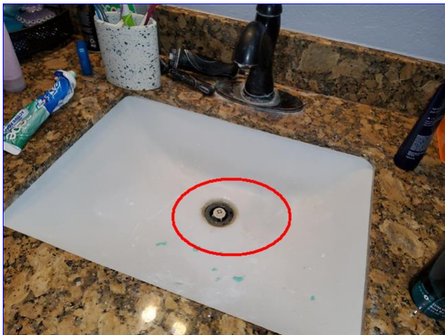
B. Item 2 (Picture) Guest bathroom
