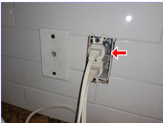
B. Item 4 (Picture) Kitchen area
