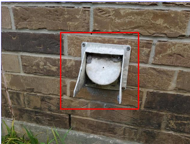
H. Item 1 (Picture) Right side
