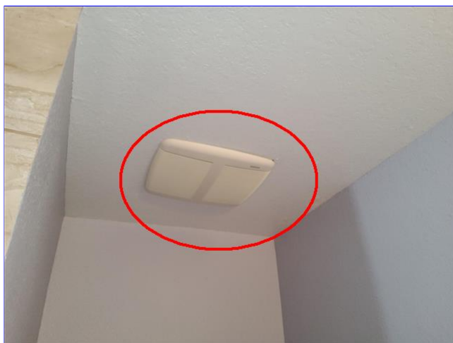
F. Item 2 (Picture) Guest bathroom
