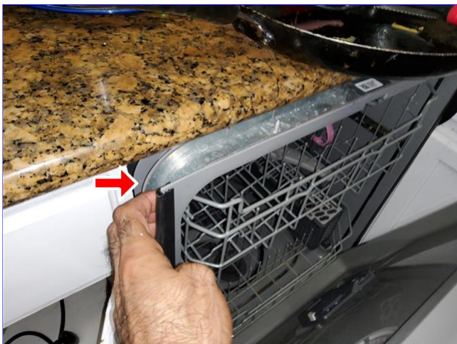
A. Item 3 (Picture) Loose/not secured
