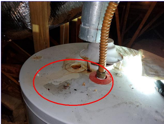
C. Item 4 (Picture) Attic Space
