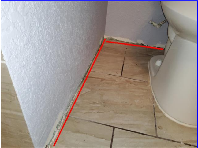
F. Item 1 (Picture) Guest bathroom
