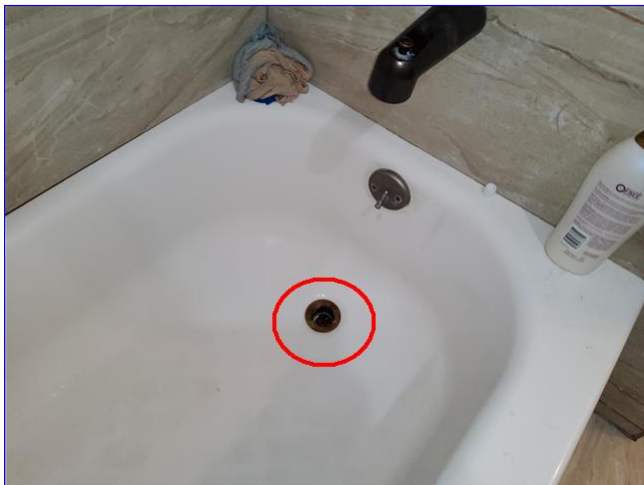
B. Item 1 (Picture) Guest bathroom
