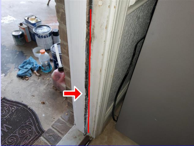
G. Item 1 (Picture) Back porch door
