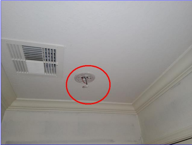
B. Item 10 (Picture) Hallway area
