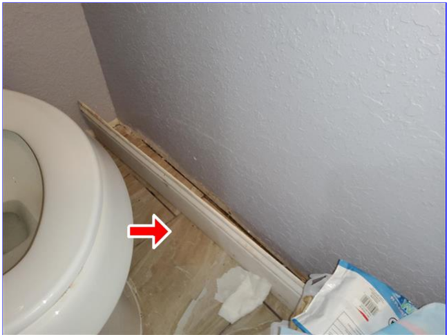
F. Item 2 (Picture) Guest bathroom
