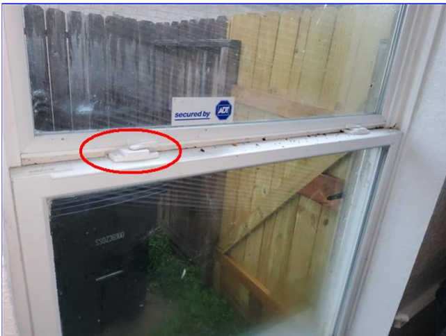
H. Item 4 (Picture) Living room area
