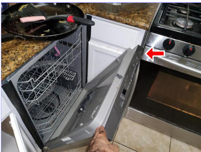
A. Item 4 (Picture) Obstruction
