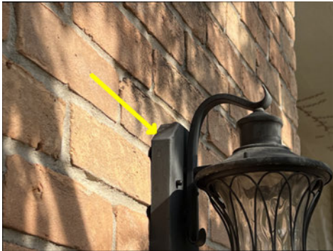
Seal all exterior penetrations.
