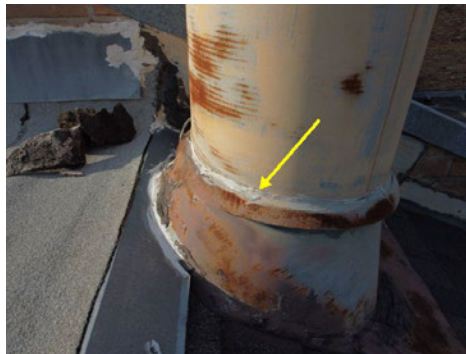
Caulk the chimney storm collar.
