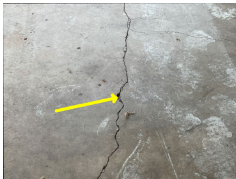
Multiple large foundation cracks observed in the garage.
