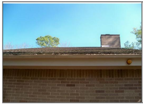
**Description:**Roof sag noted in front right roof slope
