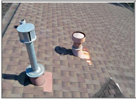
**Description:**Roof vent flashing corroded at right side
