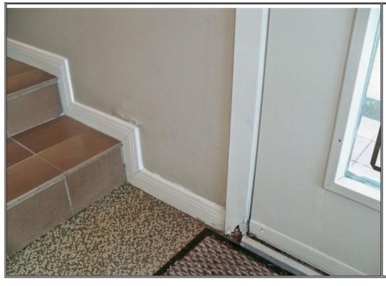
**Description:** Wood rot and water damage in gameroom wall and door frame
