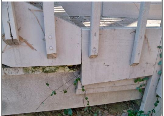
**Description:** Localized wood rot in deck stair at left rear stair to backyard
