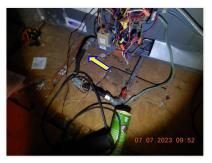
Gas supply to furnace is not installed with a sediment trap at the connection to the unit.
