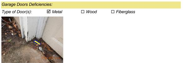
$\blacksquare$  Garage door jambs in contact with the slab surface and are damaged at some locations.
