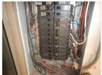
☑ The service equipment disconnecting means panel board is missing a dead front cover. INTERIOR PANEL BOARD:
