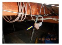
☑ Improper use of an extension cord at the following locations: Attic.
