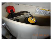
☑ The master bathroom commode flushing mechanism is damaged and not flushing properly.
