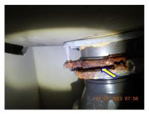
$\ensuremath{\boxtimes}$  The food waste disposal housing connection is deteriorated/rusted.
