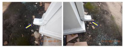
$\square$  Splash blocks should be placed in areas where water can accumulate near the foundation edge. The discharging of the rainwater from the gutters needs to be directed away from the foundation edge.
