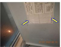
$\ensuremath{\boxtimes}$  Branch circuit service locations were not all marked at the service equipment disconnecting means panel board enclosure dead front cover.
