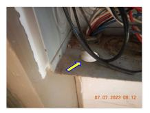
☑ One of the interior knockouts is missing at the bottom of the panel. NEUTRALS/GROUNDS:
