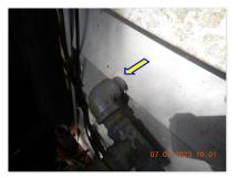
$\square$  The metal gas distribution pipe entering the building should be bonded to the electrical system. The metal gas pipe is not bonded or could not be verified at the time of inspection.
