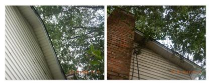
☑ The roof has tree limbs coming in close contact with the roof covering. Tree limbs can cause damage to the covering and allow access to the roof for unwanted pest. I recommend trimming back all tree limbs away from roof.
