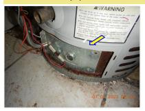
☑ Water heater control panel cover is missing.
