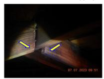
☑ Ridge boards are undersized. The ridge boards should be the depth of the rafter end cuts.
