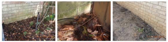
☑ High soil levels exposed under brick surfaces. DOWNSPOUTS:
