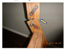
☑ Angle of the attic stairs is not properly cut, this puts a strain on the stairs. *Attic Service Access Deficiencies:*
