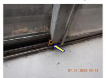
$\blacksquare$  The window at the 2nd floor back right bedroom is secured shut with a screw.
