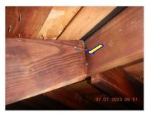
$\ensuremath{\boxtimes}$  Rafters were secured to the ridge board with 0 nails on one side, versus the appropriate number on one side, the appropriate number on the other.
