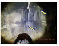
☑ Missing or deteriorated grout between firebrick at the firebox.
