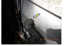
☑ The gas lines are not properly sleeved or wrapped with PVC plumbing tape where passing through the exterior veneer at the following locations: Right exterior hose bib.
