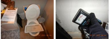
☑ Commode area- High moisture readings were noted with the moisture meter in the tested area.
