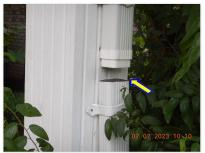
Gutter downspout pipe at the front right side of the home has a gap in it.
