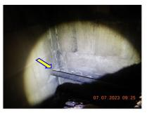
$\square$  The area where the gas line enters the fireplace should be sealed. CHIMNEY:
