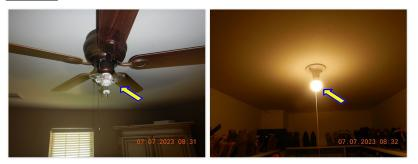
☑ Light fixture globes missing at the following locations: Garage, Master bedroom, Master closet, 2nd floor hallway closet, 2nd floor front middle bedroom closet, 2nd floor front right bedroom closet, 2nd floor back right bedroom closet, Attic.
