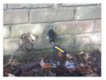
$\square$  The condensate drain line is depositing water at the exterior of the dwelling. Condensate drain line should deposit into the sanitary sewer system at a sink or tub trap.
