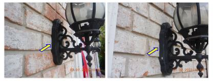
☑ Caulking/sealant is missing around the exterior light fixtures where missing/deteriorated. LINTELS:
