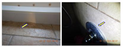
Z Caulk the bathtub/shower enclosures and around fixtures where missing or deteriorated.
