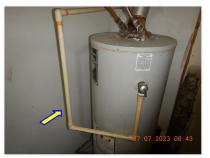
$\square$  The drain line for temperature and pressure relief valve is not installed with positive flow allowing standing water to corrode the valve.
