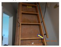
Disappearing attic access ladder ceiling panel is not insulated at the attic.
