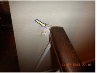
$\blacksquare$  Handrail at the bottom of the stairs is no longer secured to the wall.
