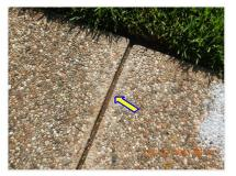
☑ The expansion joints in the driveway and walk way are open. Open expansion joints can allow water to get under the concrete surface and expand or wash away the soil causing lifting or settling of the concrete. I recommend filling the expansion joints with an approved expansion joint material.
