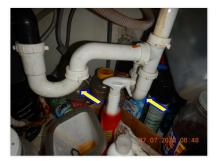
$\square$  A double P trap is installed at the kitchen sink. One P trap can pull water from the other trap and cause sewer odors to enter the home. <u>TUBS:</u>
