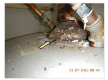
$\square$  The water heater vent draft diverter is not properly secured at the top of the unit. <u>T&P DRAIN:</u>
