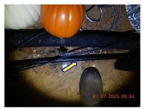
$\square$  Gas pipes and/or wires and/or water lines are crossing directly over the top of the attic service walkway.
