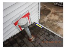
☑ Kickout flashing missing and or inadequate at some locations. ROOF JACKS:
