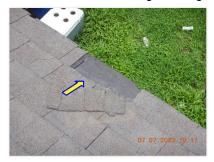
☑ Weathered and/or wind damage and/or missing shingle tabs was noted.
