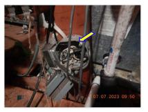
☑ Junction box cover plates observed missing at the following locations: Attic. WIRING AND CONDUIT:
