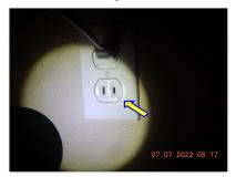
$\square$  2 prong plugs are installed at some locations. These are a type of plug that is not grounded. <u>SWITCHES:</u>
