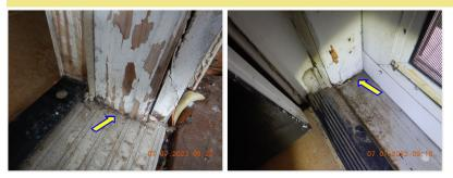
$\boxdot$  Caulking around the door missing or deteriorated. Some Examples: Front entry, Back patio, Garage entry.
