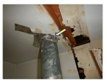
☑ Proper clearance from wood or combustible materials not installed at the water heater vent pipe. Minimum 1" clearance required for Type B vent pipe.
