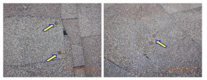
☑ Caulk face nailed ridge cap shingles where missing. <u>FLASHINGS:</u>
