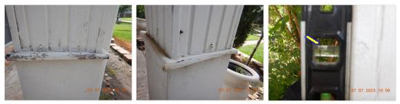
I Front patio columns are deteriorated and some are no longer level.
