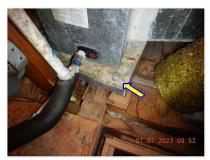
☑ Insulation/debris observed at the A/C auxiliary condensate drain pan.
