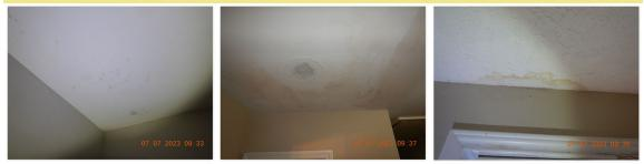
I Evidence of moisture stains observed at the following locations: 1st floor water closet, Living room, 2nd floor hallway. These were dry at the time of inspection.
