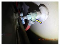
☑ Utility room washing machine bibs are corroded.
