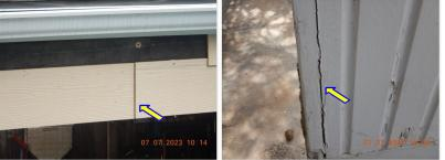
☑ Caulking is needed at all joints and unsealed seams in the siding. CAULKING:
