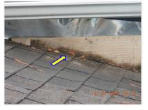
$\square$  Exterior siding is in contact with the roof. Separation between the siding and roof covering will minimize moisture entrapment and deterioration of the siding.
