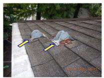
$\square$  Note: Multiple satellite dishes have been installed on the roof. Some satellite dishes and/or mounting brackets have been abandoned. These penetrations should be caulked at the fasteners. DRIP EDGE FLASHING
