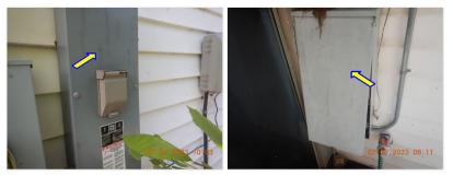
☑ The new NEC changes state that the emergency electric shut off should be labeled with a non-removable plaque.
