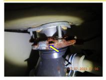
☑ The food waste disposal connection clamp is not locked into place at the sink flange. Disposal vibration may cause the unit to leak or detach at the sink connection.
