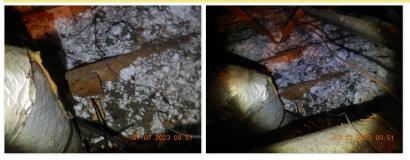
☑ Redistribute insulation where missing or moved at the attic floor.
