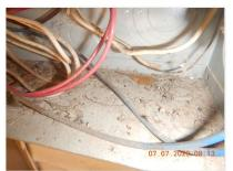
$\ensuremath{\boxdot}$  Debris observed at the interior of the service equipment disconnecting means panel board enclosure.
