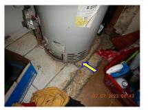
☑ No drain pan is installed under the water heater. INSTALLATION:
