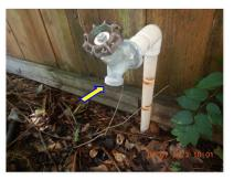
☑ Exterior hose bibs not installed with anti-siphon devices at some locations. <u>SINKS:</u>
