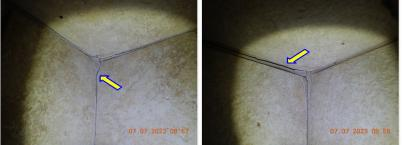
$\blacksquare$  Mortar is cracked at the the master bathroom shower enclosure.
