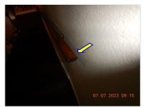
☑ Stairway hand railing ends should terminate into the wall or newel post.
