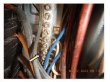
☑ Ground wires are double terminated. There should be one ground wire per screw terminal. CIRCUIT BREAKERS:
