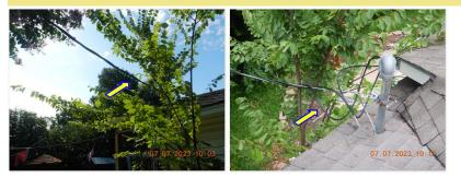
$\blacksquare$  Service entrance conductor does not have proper clearance from the walking surface and roof covering.
