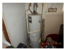
$\blacksquare$  The water heater is installed in a prohibited location. Excess combustible fumes can enter the home.
