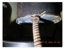
$\square$  The food waste disposal whip cord is not properly secured at the clamp at the base of the food waste disposal.
