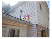
☑ The water heater vent pipe terminates within 8 feet from vertical wall or eave at roof level.
