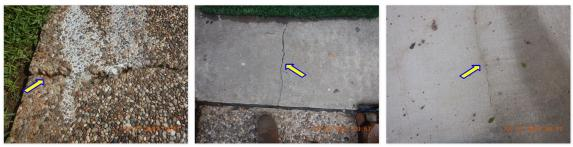
☑ Settlement cracks observed at the flatwork at the following locations: Front walkway, Driveway, Front patio, Back patio.
