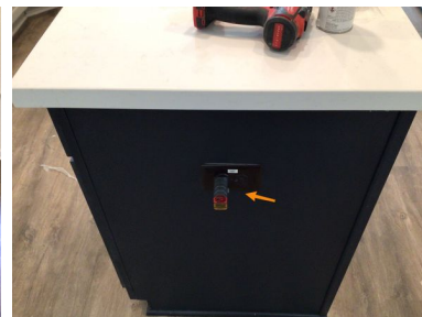
Multiple Locations in Kitchen
