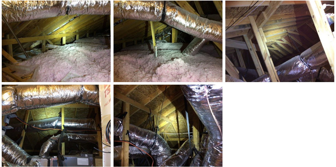
General Photos of Structure:
