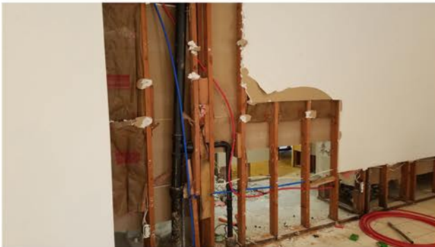
Installation of PEX plumbing throughout the house.
