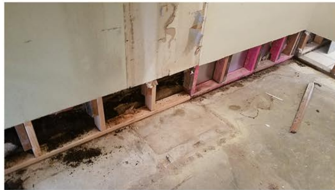
Replacement of all rotten wood inside interior walls
