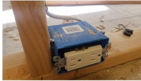
Update of electrical panel, outlets and electrical safe boxes
